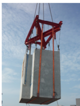
Lifting PBU in place
