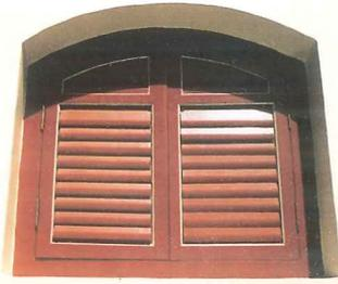
*Arched window shutter with fixed and openable louvres matching the original*
