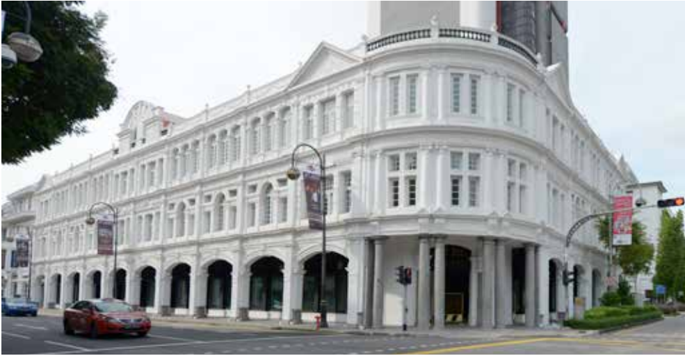
Stamford House returned to its original use as a hotel
