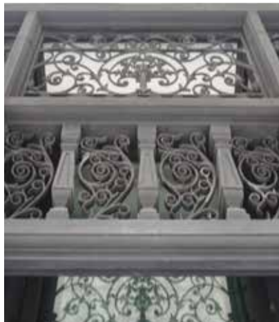
Cast iron and timber shopfront details
