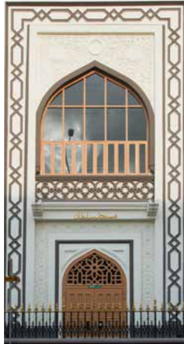
Original woodwork retained
