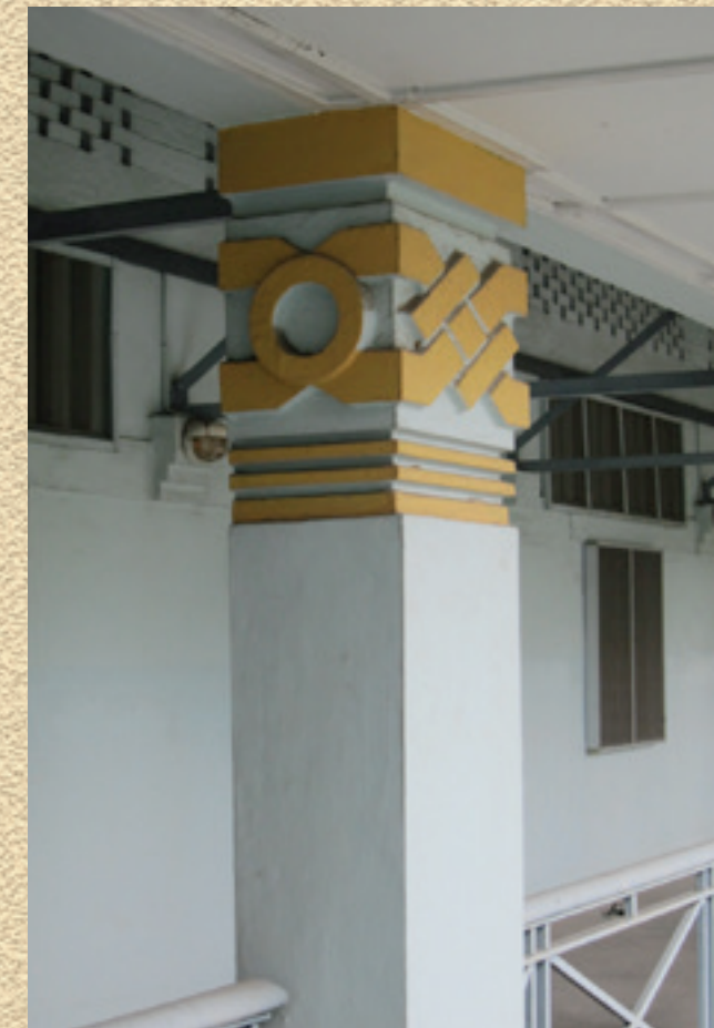
Art-Deco style motif on the column capitals
