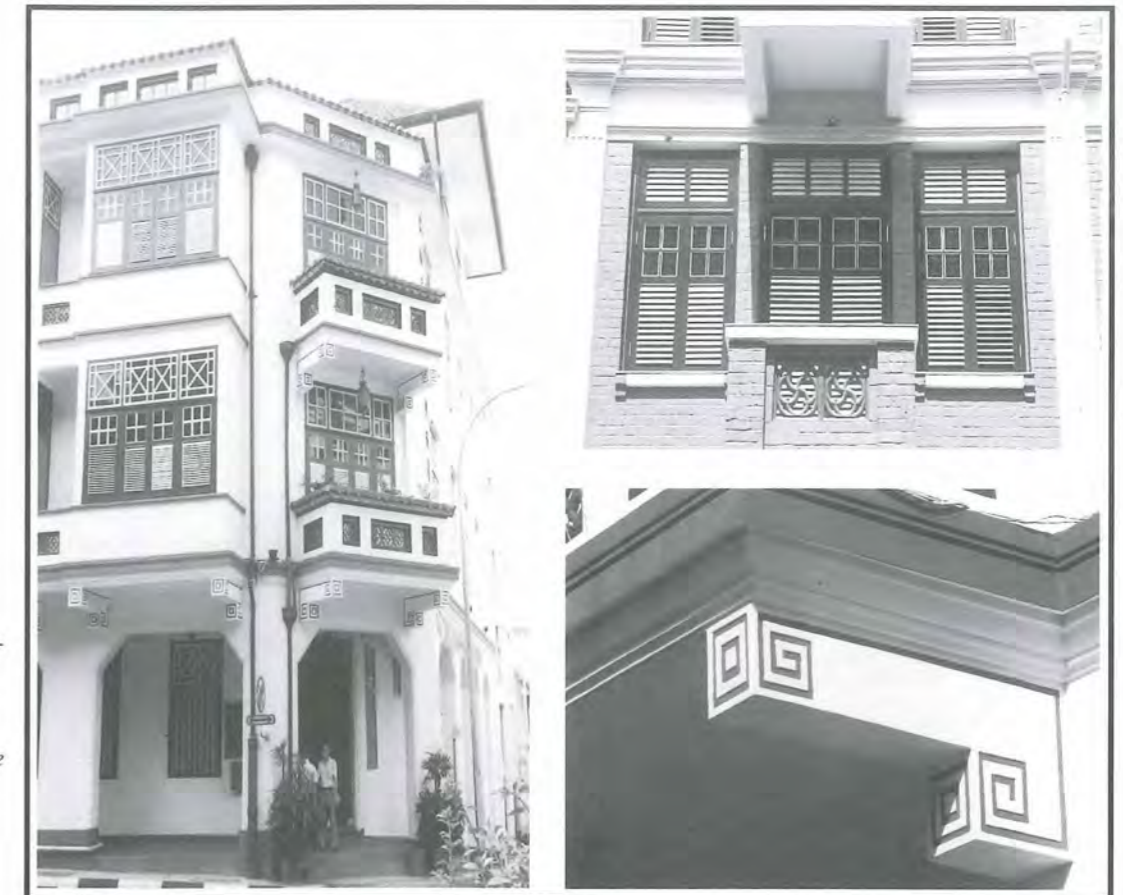
Fig 6: The Art Deco Style (1930-1960) is typified by the streamlining of classical motifs such as capitals, arches and keystones. The use of simple-designed corbels and fair-faced bricks are common features.
