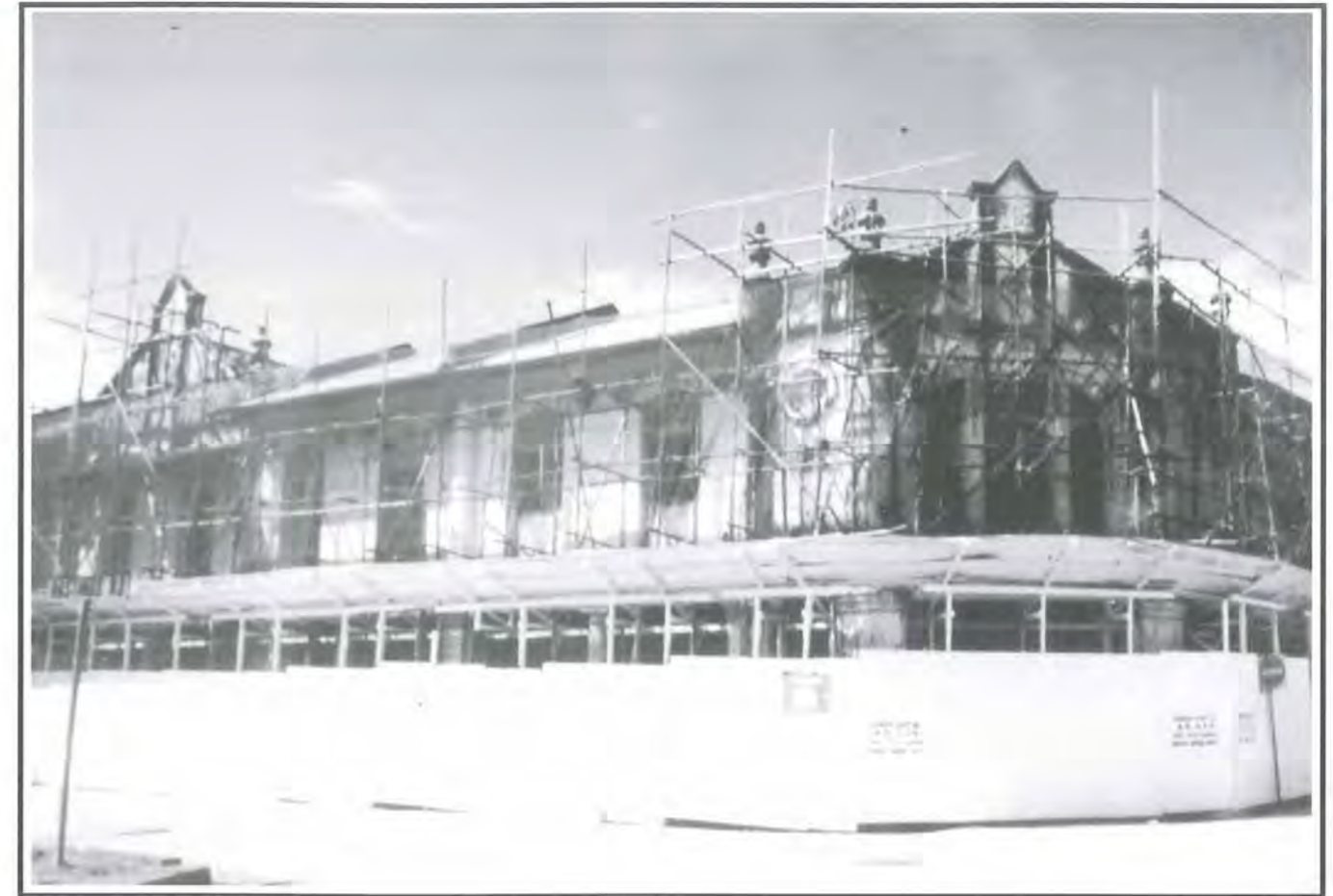
Fig 15: Temporary hoarding is required during the restoration works. This not only protects the elements from further deterioration and collapse, but also acts as a safety measure to prevent accidents.
