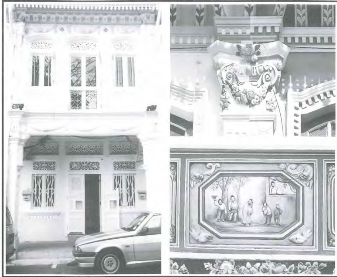
Fig 4: The Late Shophouse Style (1900 - 1940) is the most spectacular, especially in the use of ornamentation. Brightly-coloured ceramic tiles and plaster bouquets, festoons, plaques and other elaborate ornamentation are evidence of the builder's artistry.
