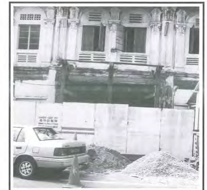
Fig 17: Temporary propping of facade walls to prevent collapse during restoration.
