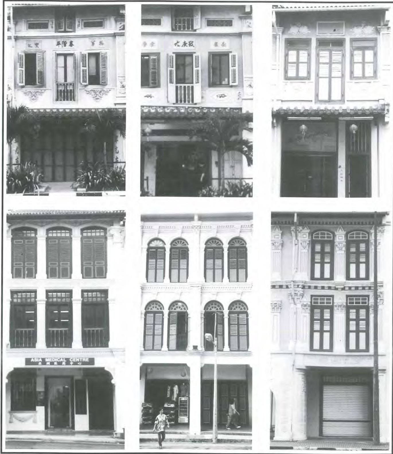
Fig 43: Restored facades where the original ornamental mouldings and features are retained. They enhance the historical significance of the conservation buildings.
