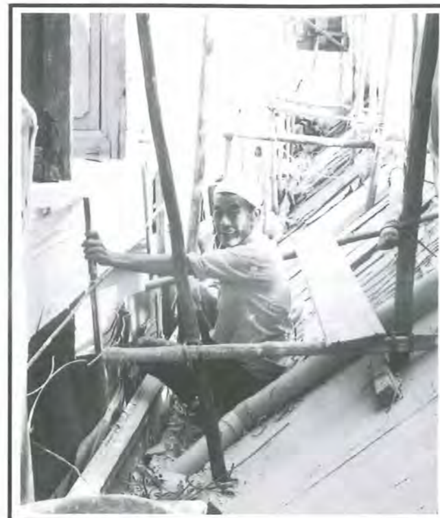
Fig 14: Temporary hoarding set up for restoration works to be carried out.
