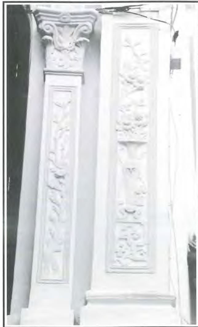
Fig 8: The loss in clarity and sharpness of the relief mouldings on the columns as a result of several layers of paint applied over time.
