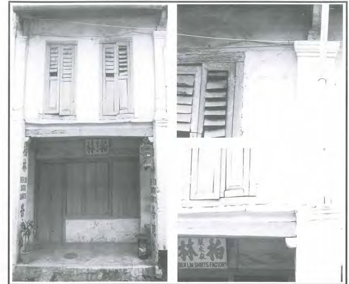
Fig 2: The Early Shophouse Style (1840 - 1900) has minimal ornamentation. Cornices and horizontal mouldings along the beams and columns of the Tuscan and Doric Orders are the types of ornamentation adopted for these shophouses.
