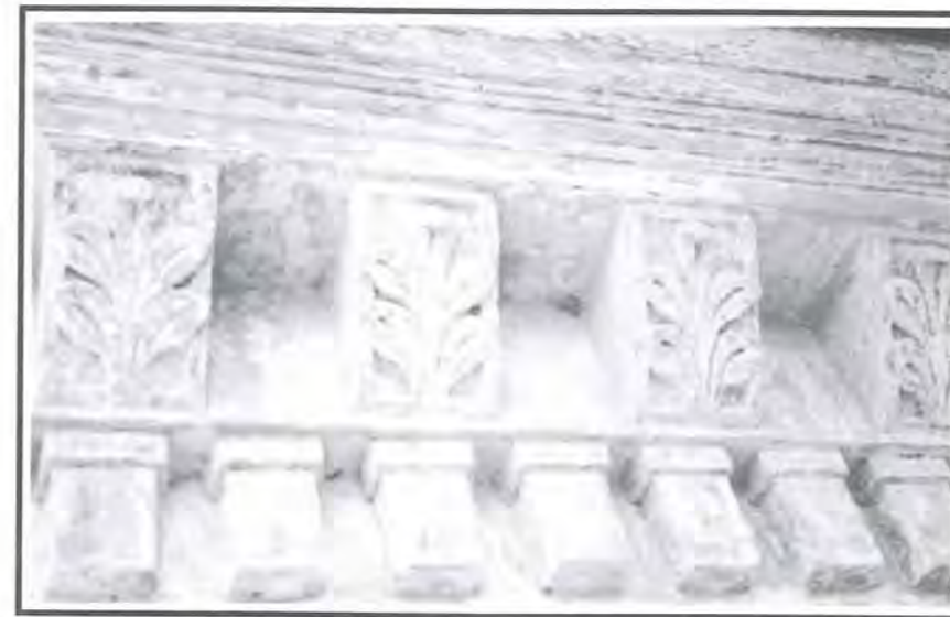
Fig 36: Surface properly cleaned and prepared for repainting.
