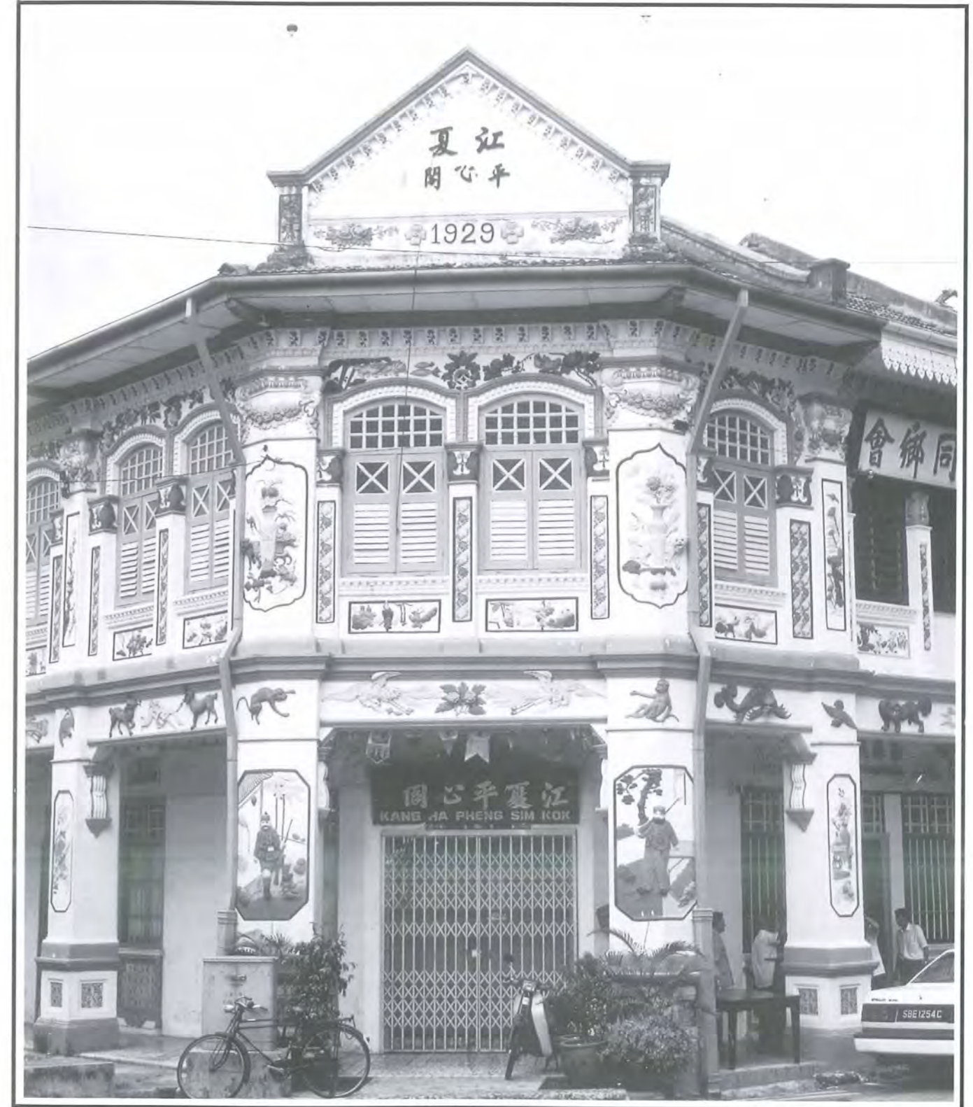
Fig 44: The historic integrity and significance of the conservation building is retained and enhanced by the well-restored plasterworks, which are characteristic of the period in which the building was built.
