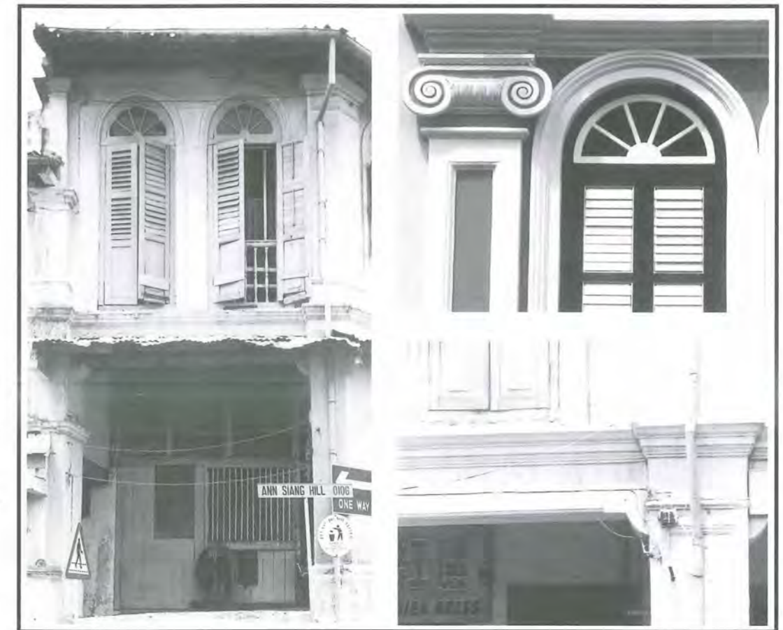
Fig 3: The First Transitional Shophouse Style (Early 1900s) usually has a lighter expression due to the greater height of each storey. Transoms are flat-arched or semi-circular and infilled with carved timber panels. The use of cornices, dentils and upturned string courses give an overall expression of elegant simplicity.
