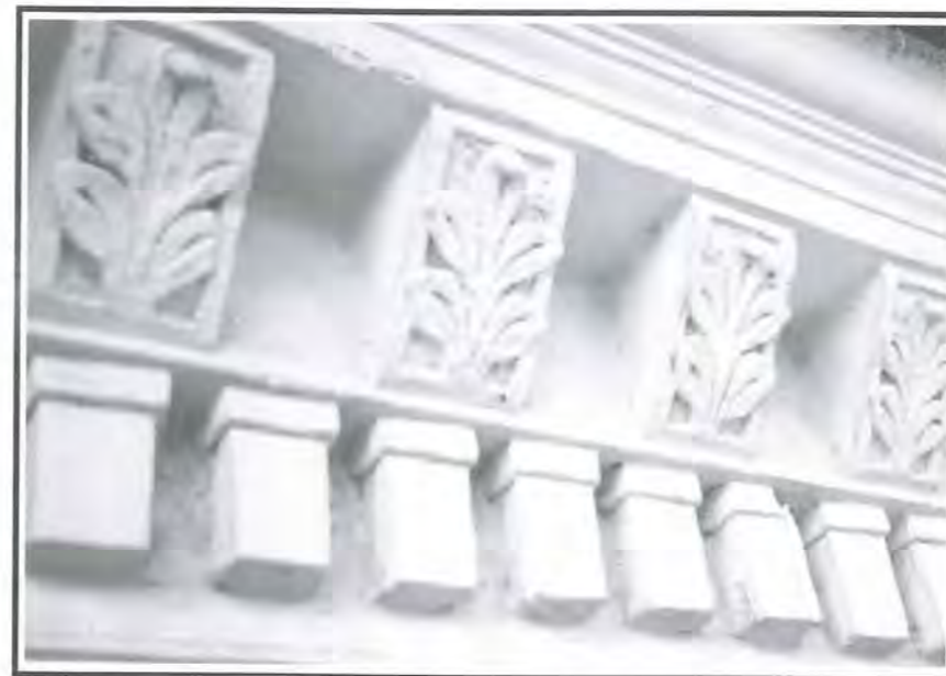
Fig 37: Repainted ornamental plasterworks.
