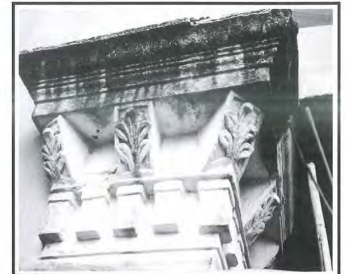
Fig 13: Deteriorated column capital due to improper detailing, water penetration and accumulation of environmental grime. This indicates the need for cleaning and repair works.
