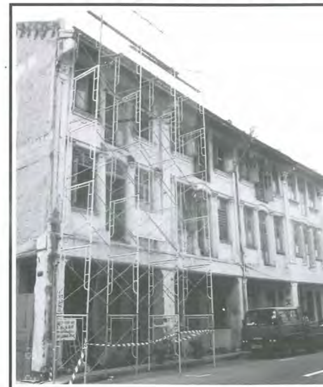
Fig 16: Temporary scaffolding and protective covering to be put up to protect the facade elements during restoration.
