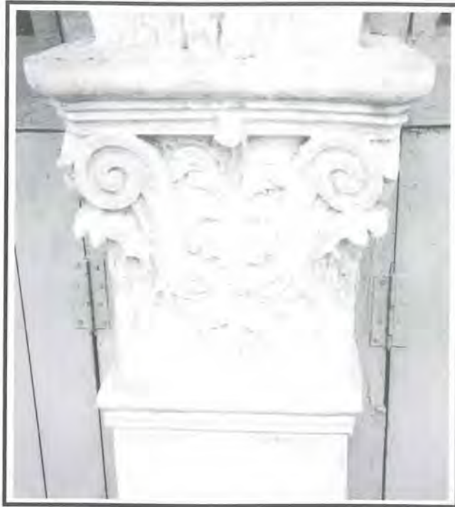
Fig 19: Cleaned plasterworks revealing the intricate details, otherwise covered by excessive paintworks.
