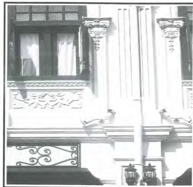
Fig 34: Intricate details properly reinstated and repainted upon restoration.
