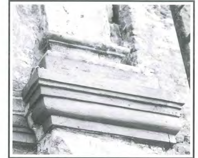
Fig 30: Repaired capital of column on the front facade.
