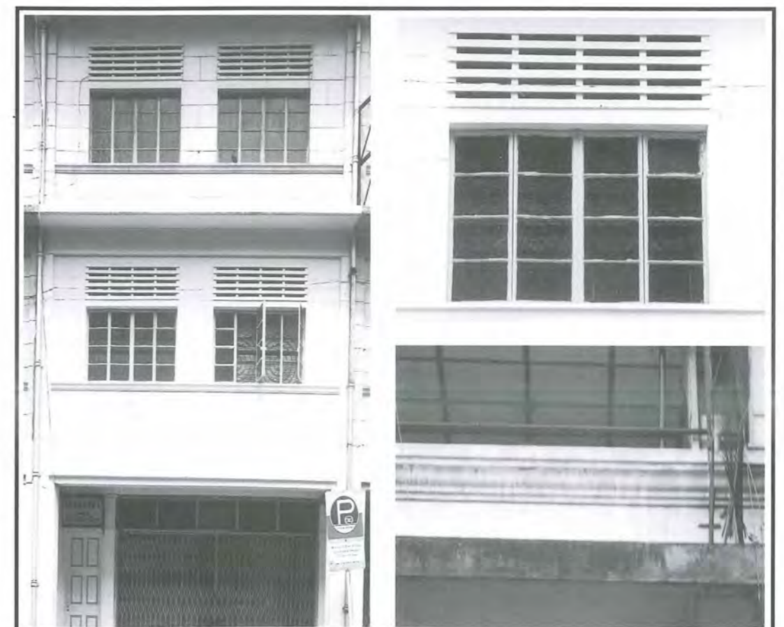
Fig 7: The Modern Style (1960s) is characterised by a geometric, free-form approach. Overhanging concrete sunshading fins, use of rustication and rectangular-shaped concrete transoms, are common features of this style.
