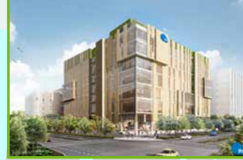
Woodlands North Coast Building 1
