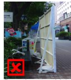
Exposed counterweight/ sandbags & brackets
