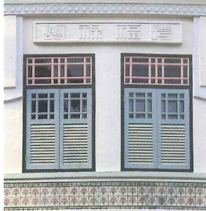
Traditional signs or characters found in plaster relief above windows
