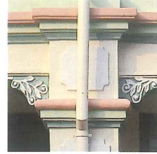
Rainwater downpipe sensitively integrated with existing column
