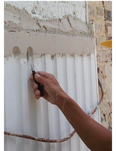
Judicious repair of plaster by craftsmen
