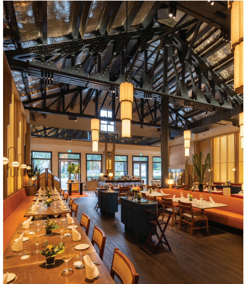
Exposed roof trusses crown the expansive internal spaces
