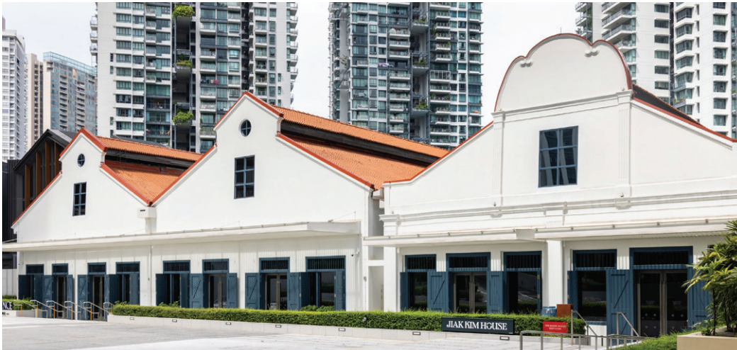
Sensitive additions and meticulous restoration breathe new life into historic warehouses
