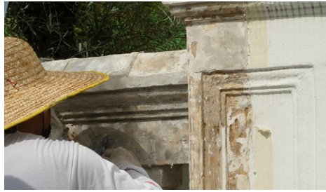
Skilled expertise engaged throughout in the cleaning and repair of original elements such as the plaster and timber work
