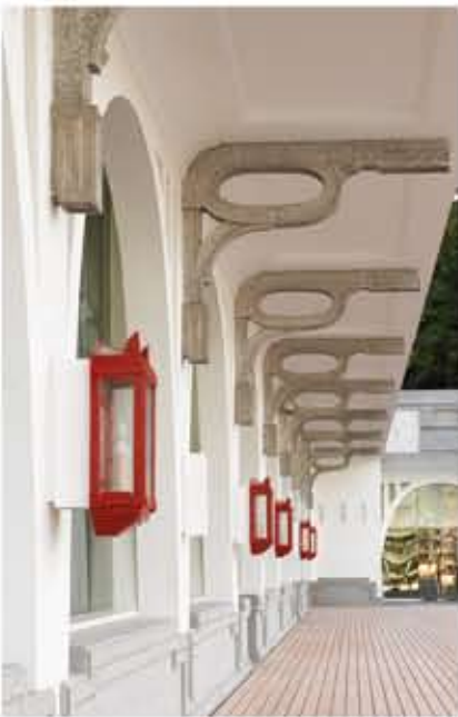
Characteristic Architectural Elements of Clifford Pier
