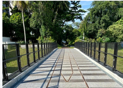
Railway tracks embedded into the flooring of the new Hillview Bridge to reflect the function of the original bridge as a railway crossing
