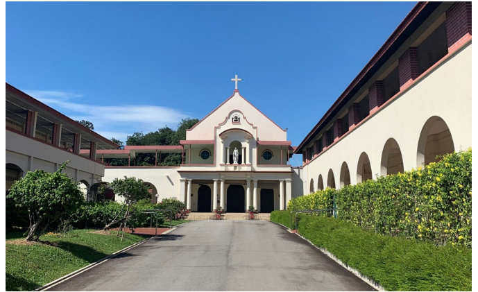
The conserved buildings at St. Theresa's Home include the Chapel, Administration Building (on the right) and Sisters' Quarters (on the left)
