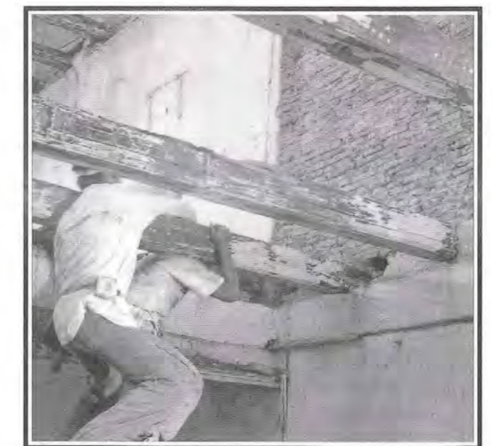
Fig 14: The replacement of the decayed timber floor joists.
