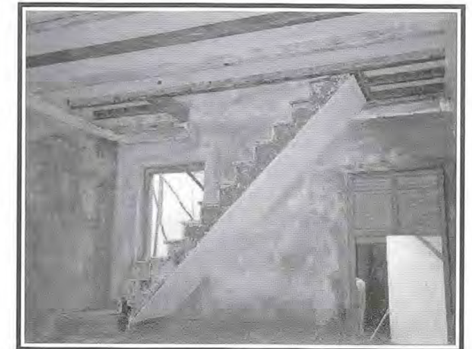
Fig 3: Timber floor and staircase in the process of being restored.
