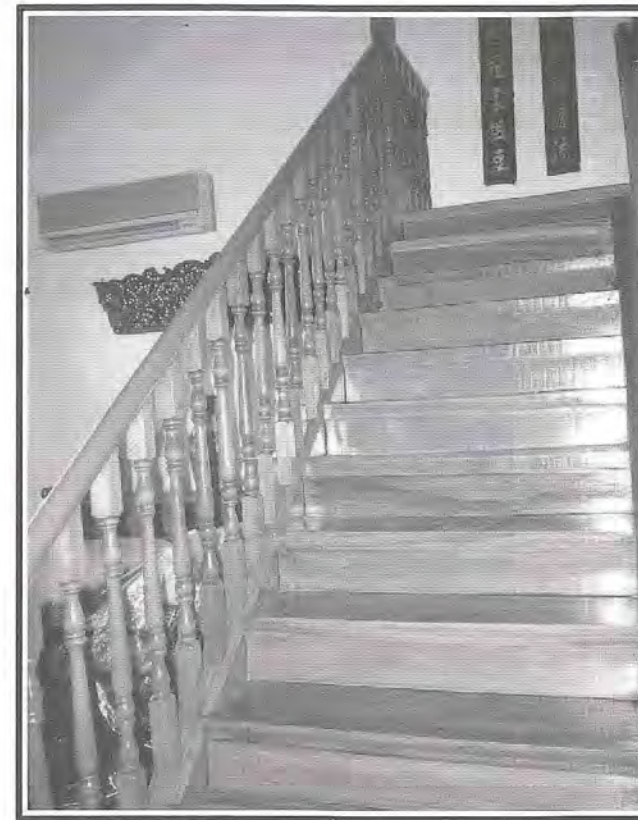
Fig 18: Timber staircase reconstructed to comply with current building codes.
