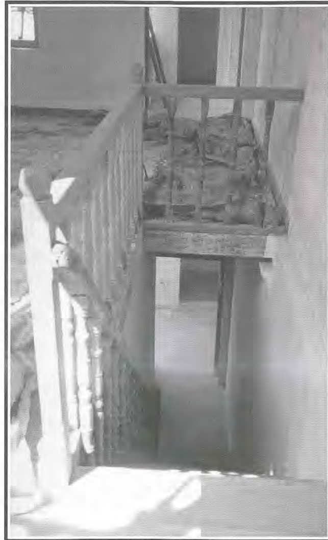
Fig 17: Restored staircase, using matching balustrades.
