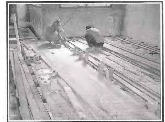
Fig 22: The laying of the new fire-retardant timber boards.
