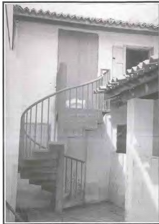
Fig 25: New metal spiral staircase at the rear court.
