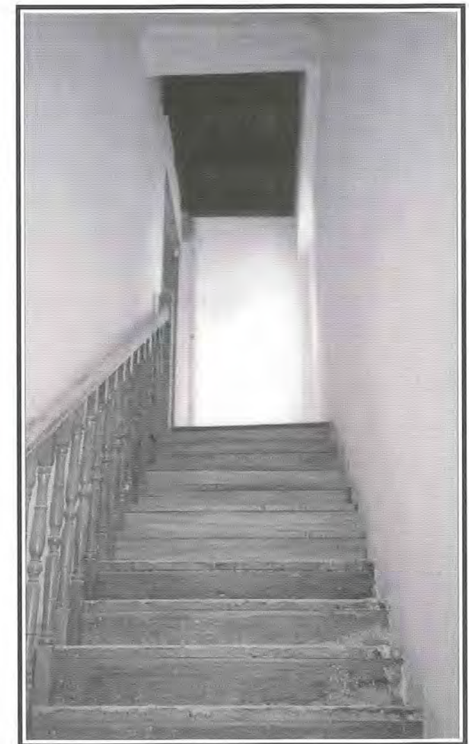
Fig 28: A completed compartmentalised staircase.
