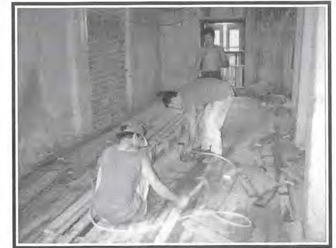
Fig 22: The laying of the new fire-retardant timber boards.
