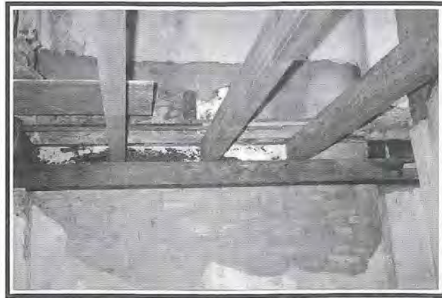
Fig 9: Repairs at the connections between timber joists and the partywall.
