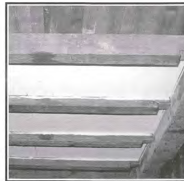
Fig 13: Use of galvanised steel brackets at the repair joints.
