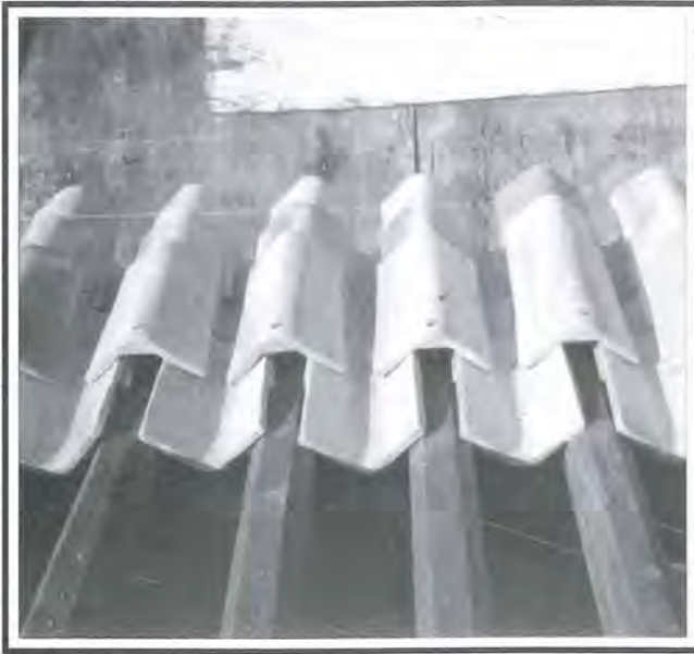
Fig 16: The use of galvanized nails properly sealed with silicon for fastening the tiles onto the trapezoidal battens.
