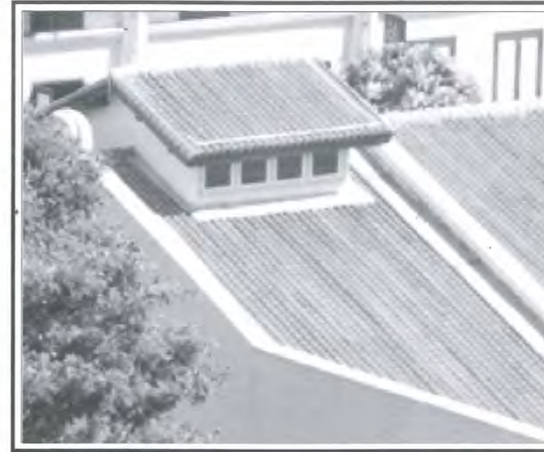
Fig 2: The double-pitched jackroof with roof tiles similar to that of the main roof.
