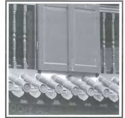
Fig 3: The ornamental green glazed canopy at the front facade is a traditional feature of the shophouse.
