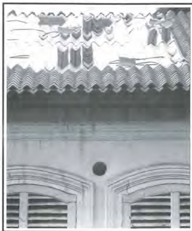
Fig 13: The laying of the tiles on the primary metal decking roof.
