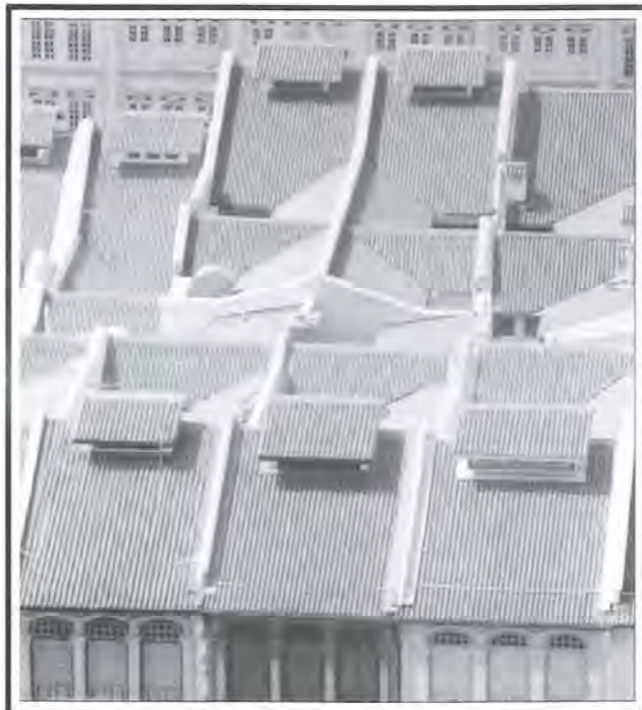
Fig 21: The firewalls also contribute to the scale and texture of the roofscape in conservation areas.
