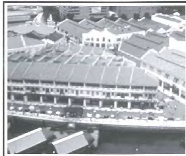
Fig 26: The restored roofscape in Clarke Quay.
