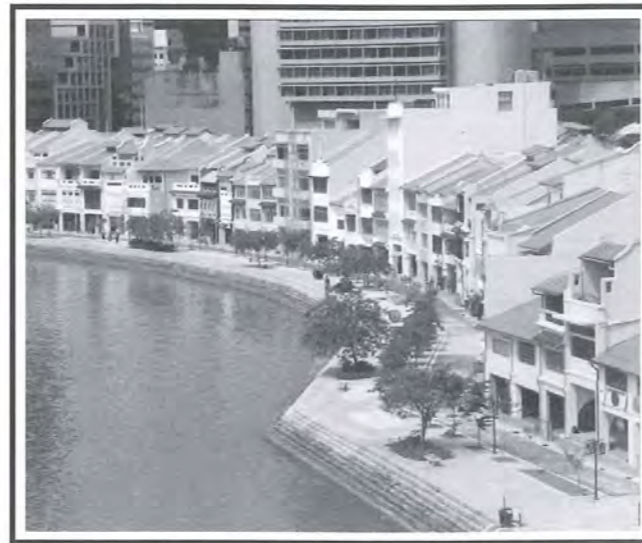
Fig 25: The restored roofscape in Boat Quay.
