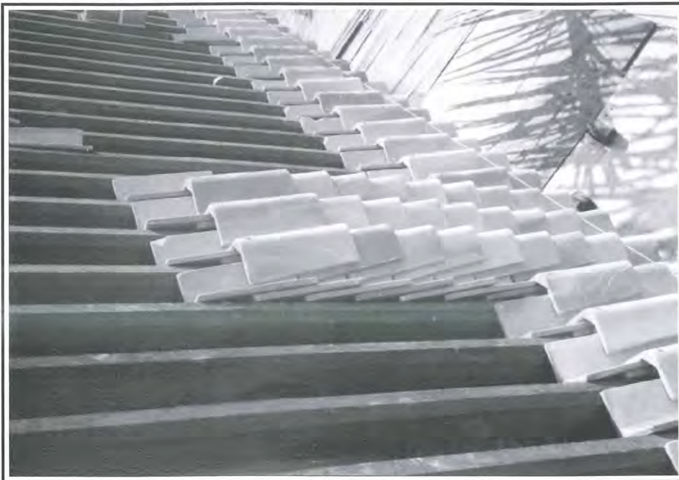
Fig 17: The use of trapezoidal battens and longer tiles for better overlap.
