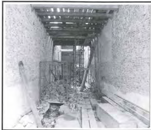
Fig 31: The partywalls during restoration.
