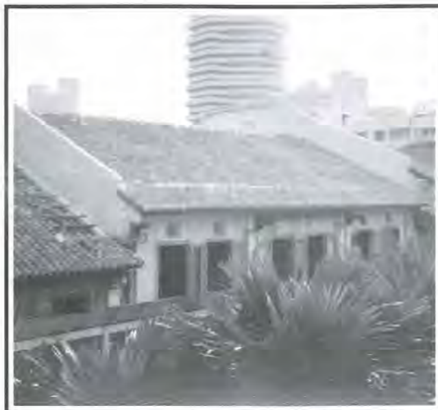
Fig 25: Shophouse units where firewalls do not protrude above the roof.
