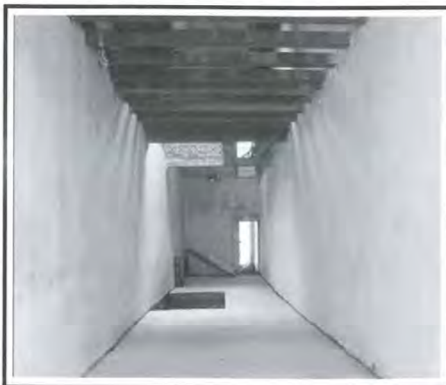
Fig 32: The partywalls after restoration.
