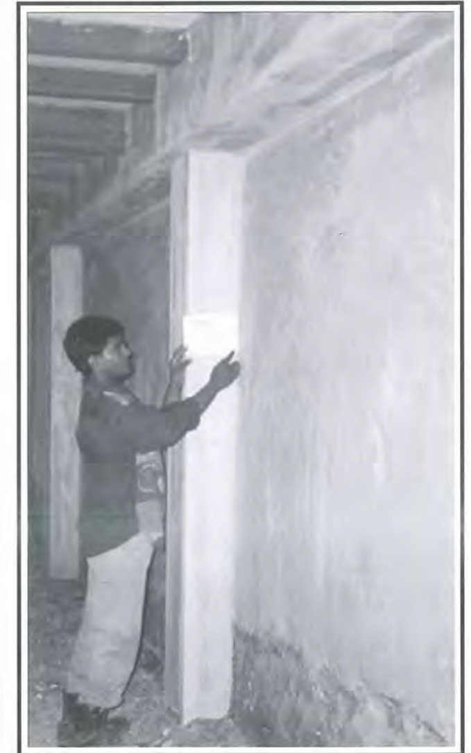
Fig 18: The new coats of plaster rendering applied to the wall
