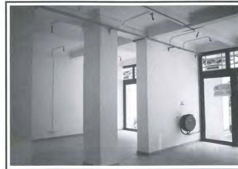
Fig 34: The structural integrity of the old building reinforced with the use of reinforced concrete structures.
