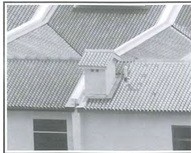
Fig 13: New flues on the rear slope of the secondary roof.
