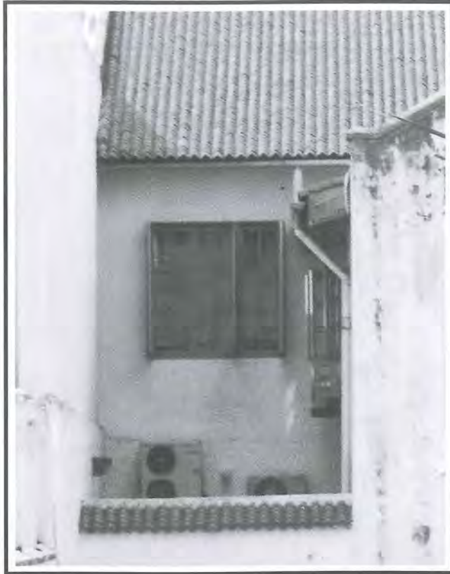
Fig 5: For buildings without roofs over the rear courts, the air-conditioning units should be installed within the rear courts such that they are least visible from the exterior.
