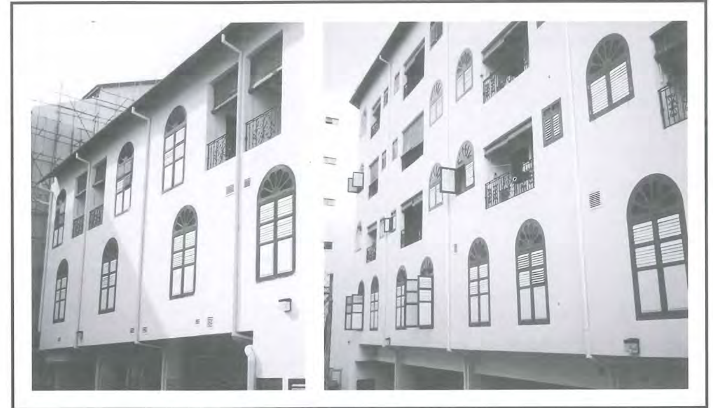
Fig 7: For projects with 3 or more connecting shophouses without rear courts, the rear of the shophouses could be modified to create balconies. The condensing units can then be located within the proposed rear balconies.
