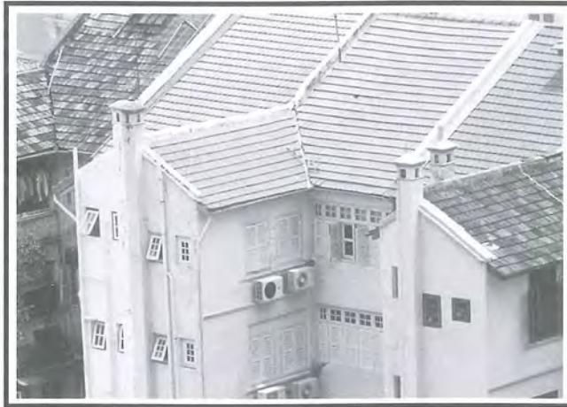
Fig 11: Existing flues abutting the rear service blocks of conservation buildings.
