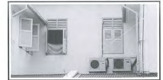
Fig 10: The ducting from the compressor units is well concealed within the casing which has been painted to blend with the wall of the rear service block.
