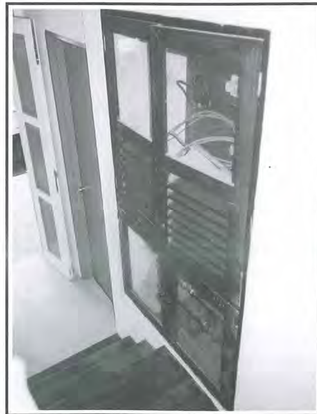
Fig 1: Electrical and water meter compartment boxed up with metal louvred casing.
