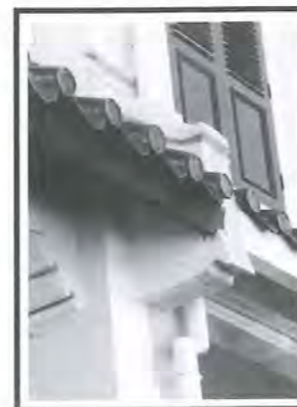
Fig 14: Corbels support the canopies at the 2nd storey floor level.
