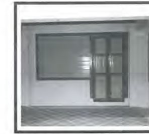
Fig 17: Traditional shopfront with demountable timber shutter boards.
