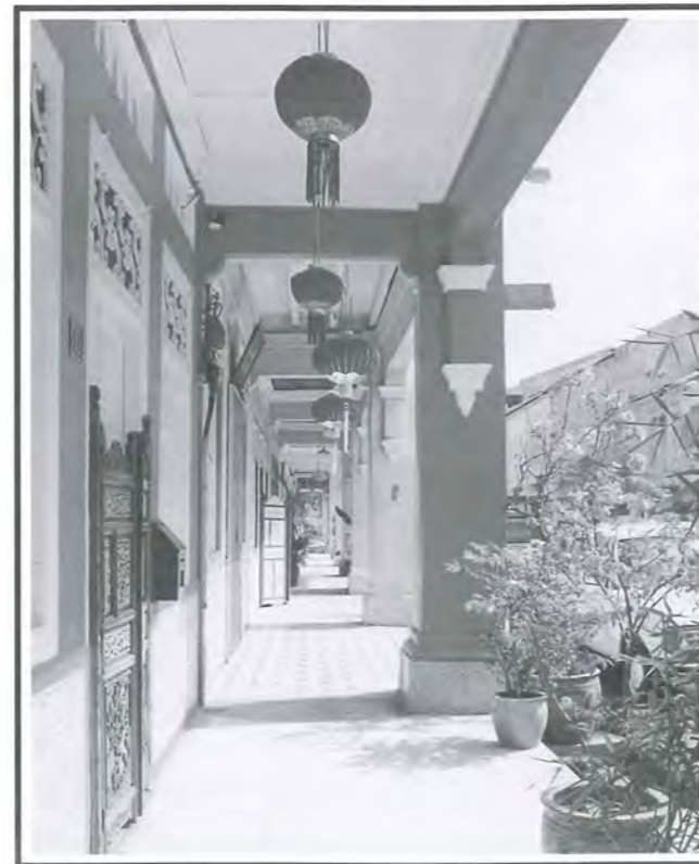
Fig 5: The key elements of the five-footway: the floor, the ceiling, the colonnade and the residential front, contribute to its traditional character.
