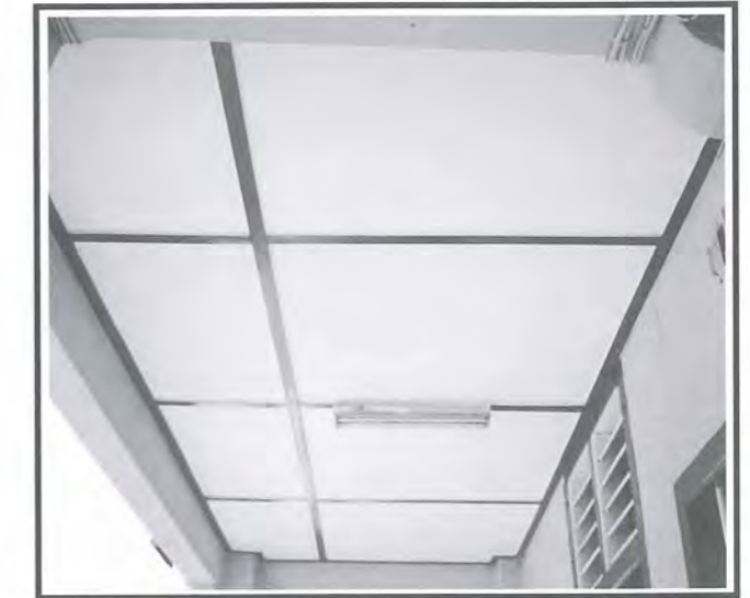
Fig 12: Ceiling of painted timber frame with cement-board finish.
