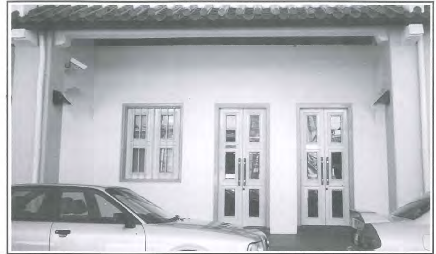
Fig 34: In facilitating a residential front for commercial adaptive reuse, timber-panel infills of the timber framed casement windows and doors are replaced with glass infills to allow for more visibility into the interior.
