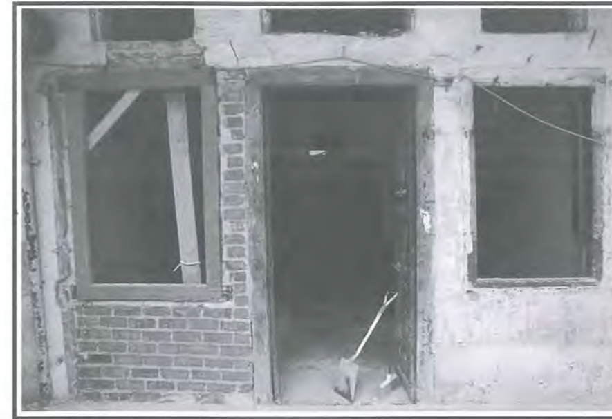
Fig 26: Part of a deteriorated residential front being replaced.
