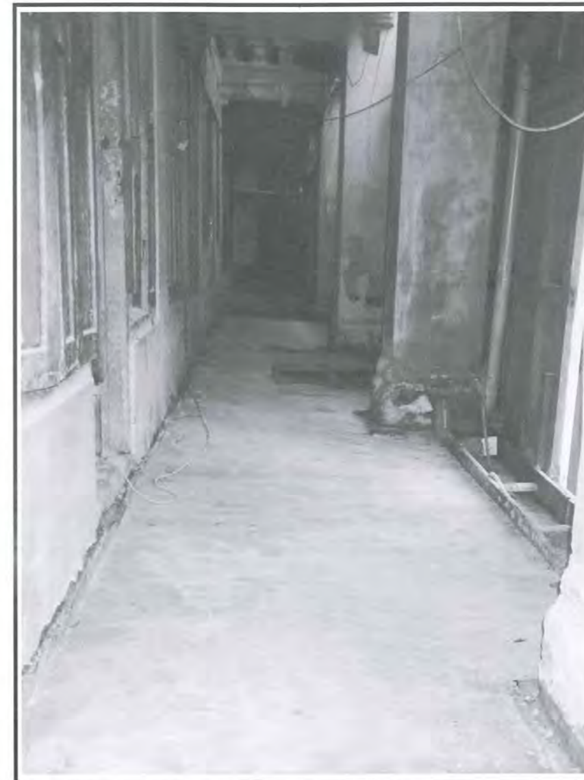
Fig 33: Ground slab of five-footway completed.
