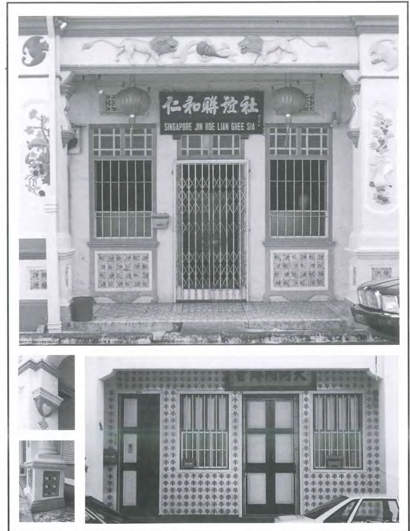
Fig 6: Examples of ornamental plasterworks and polychromatic embossed tiles found on walls and columns at the first storey.
