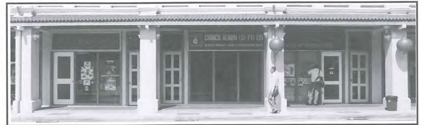
Fig 3: A variety of shopfront designs at the first storey reflecting the mix of retail shops/offices/leisure establishments within a streetblock.
