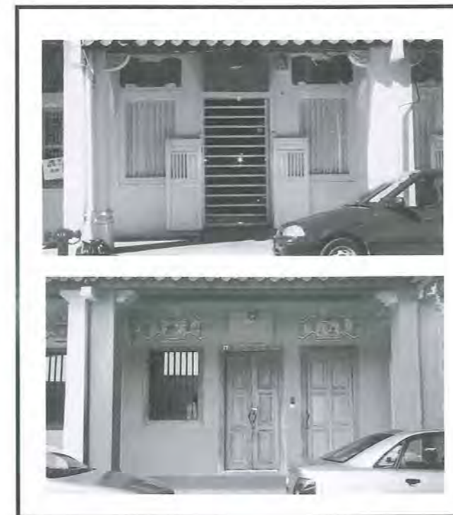
Fig 16: Residential fronts are characterised by a double-leafed timber door with a pair of timber casement windows on either side. Residential fronts which are adapted for commercial uses have two double-leafed timber doors and a timber casement window.
