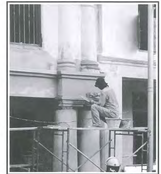
Fig 29: Restoration of column capital in progress.
