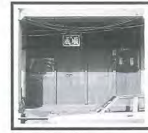
Fig 19: Traditional shopfront of double-leafed timber shuttered doors.
