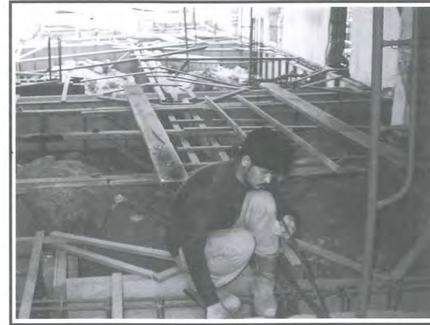
Fig 32: Reconstruction of the ground slab in progress.
