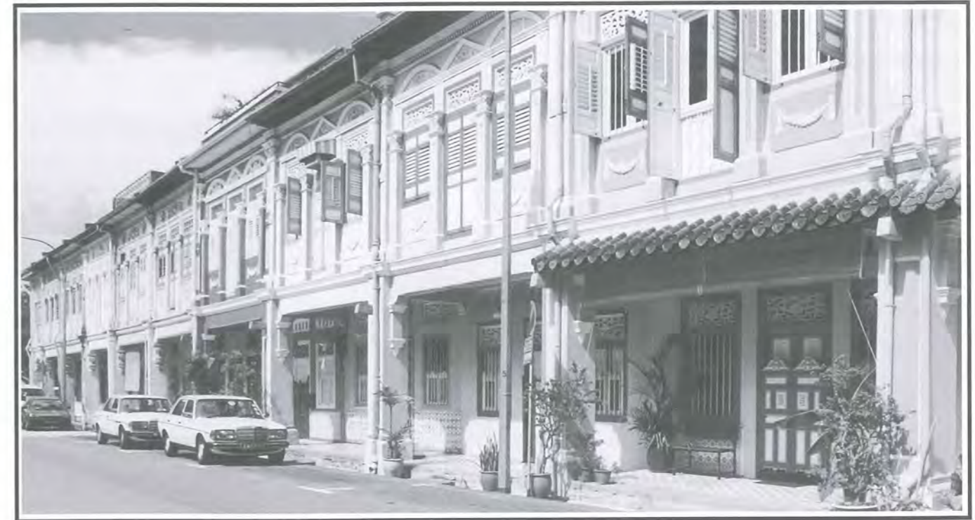
Fig 2: The five-footway is one of the key features of the shophouse. It forms a continuous walkway at the first storey.
