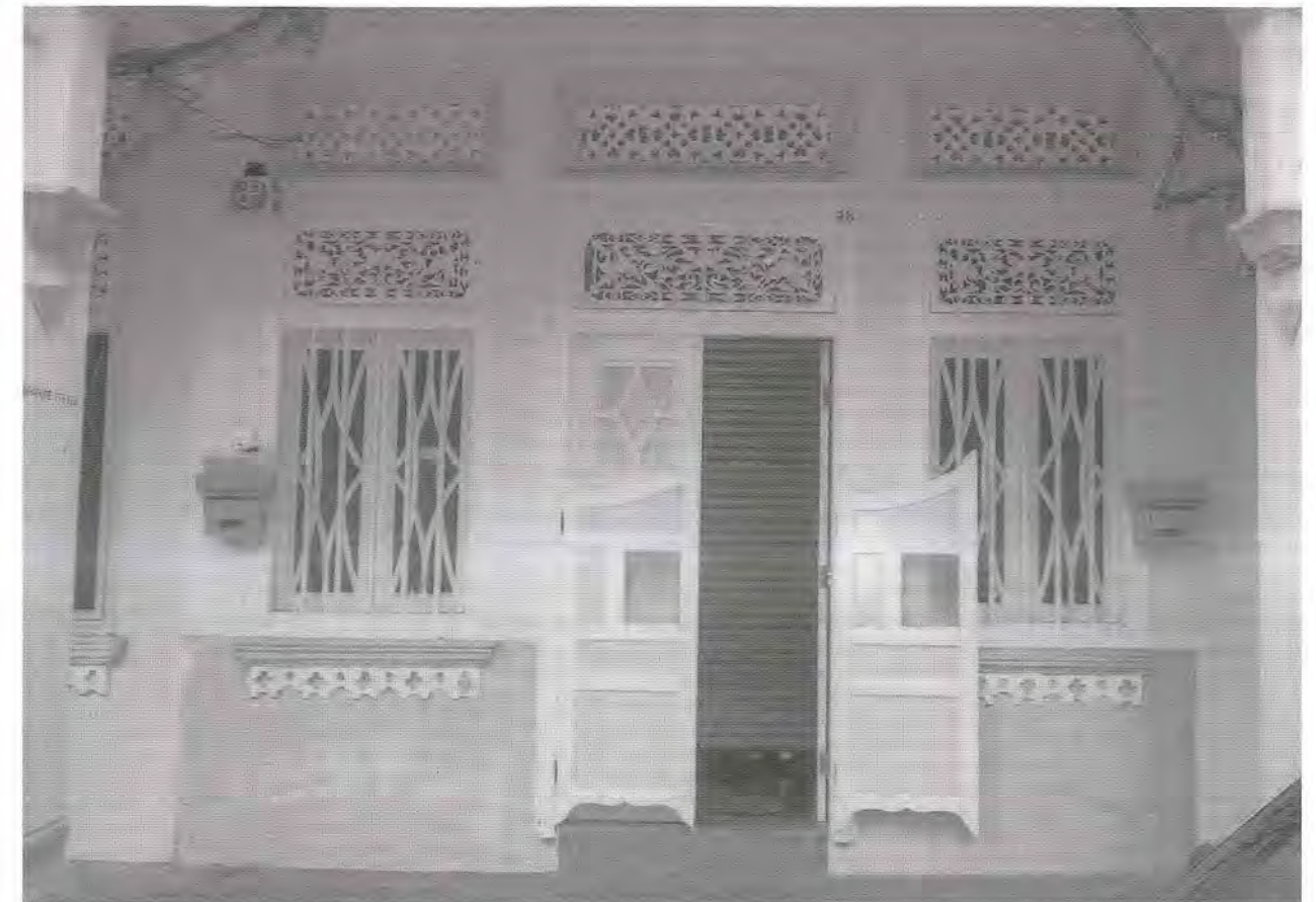
Existing elements when well-maintained reduces the need for total replacement. Regular thorough maintenance will prolong the service lives of the doors, windows and vents which have been pains-takingly restored.
