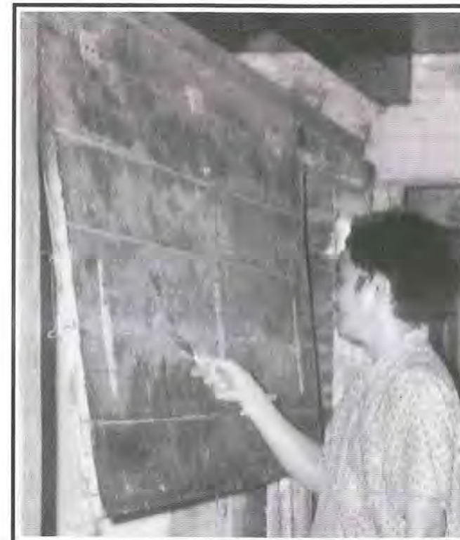
Fig 5: Scraping off the painted surface of the panelled shutters.
