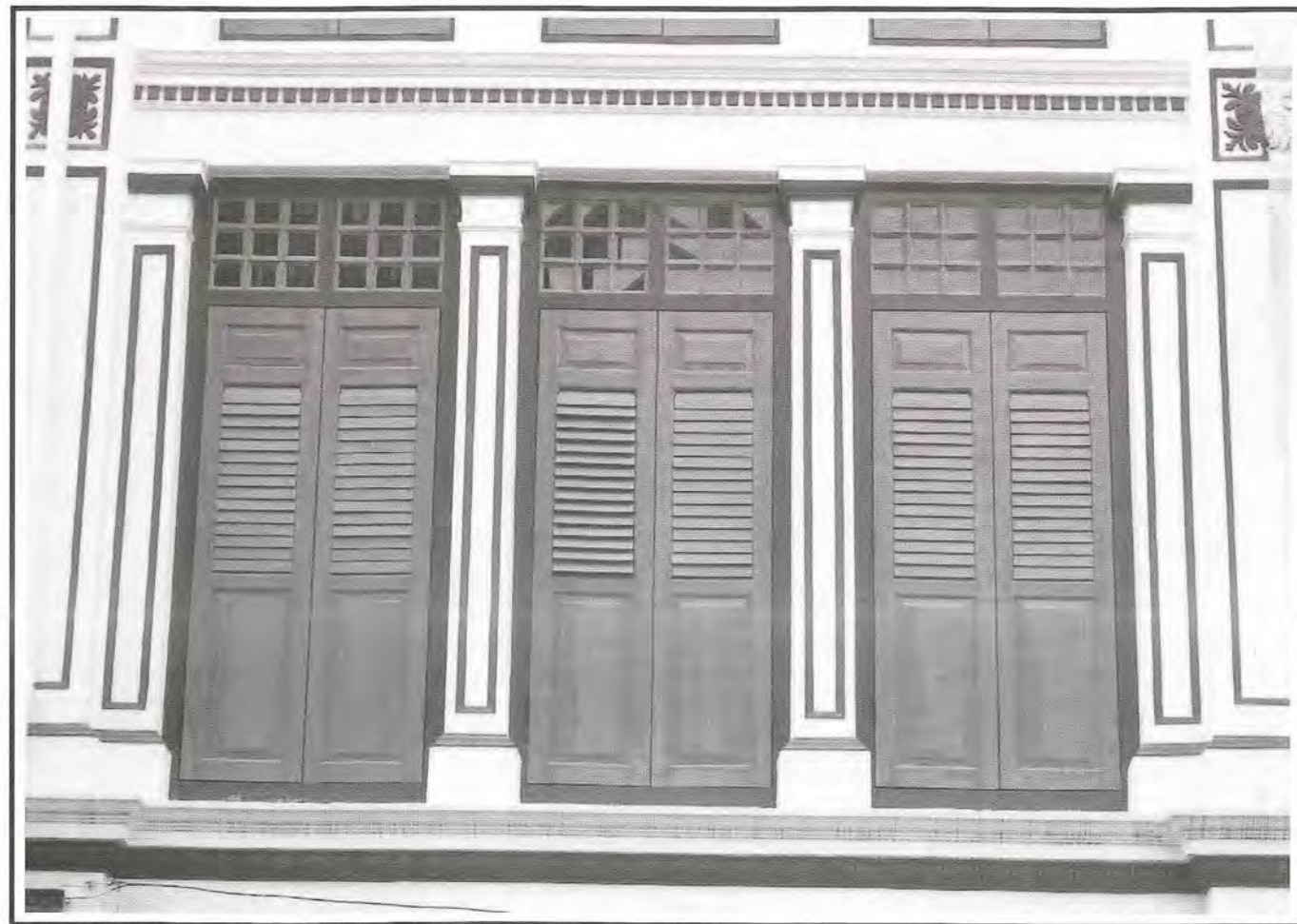
Fig 12b: After restoration Repainting to define and accentuate the French windows and architectural features.
