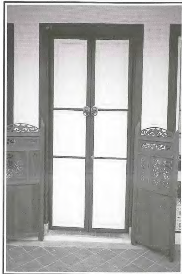
Fig 18: Restored timber panelled entrance door with decorative pintu pagar.
