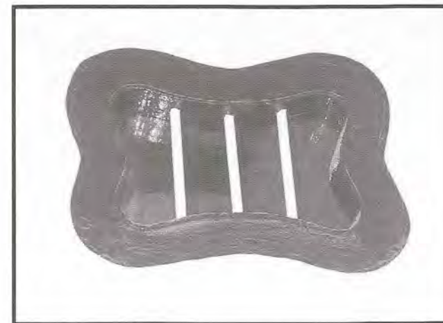
Fig 17 Top: External view of bat-shaped vent. Bottom: Internal view of the vent with glass infill to adapt to modern air-conditioning.
