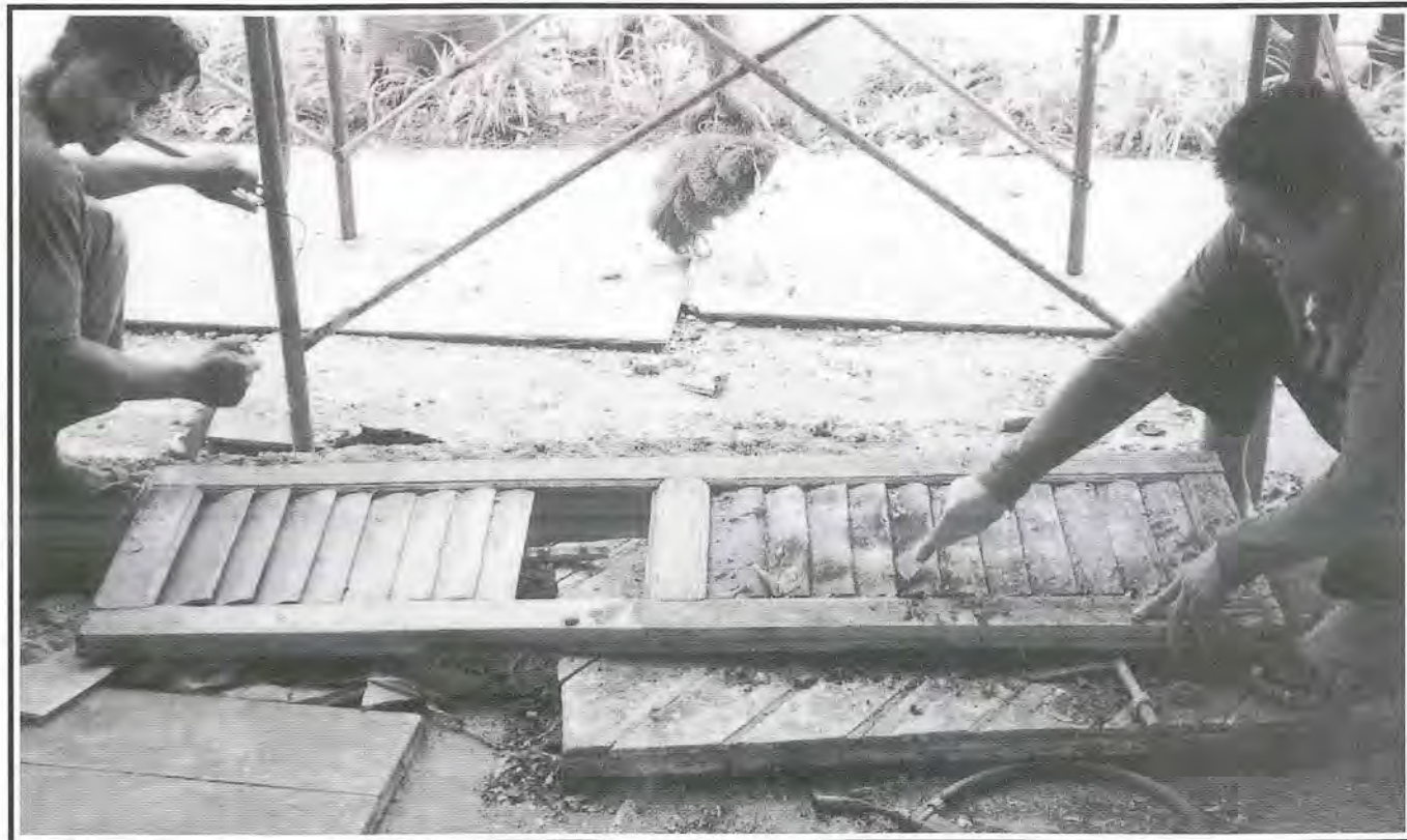
Fig 7: Preparing the surfaces of a timber louvred window.
