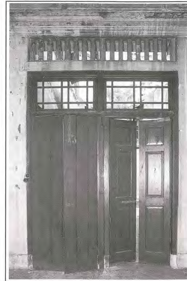
Fig 3: Eroded door panels on site. The rail and stile panels on the left should be replaced with matching timber panelled doors during restoration.
