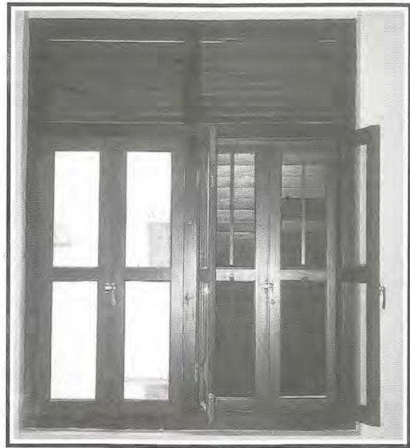
Fig 15: Intermediate rails of secondary windows matching those of the original casement and French windows.
