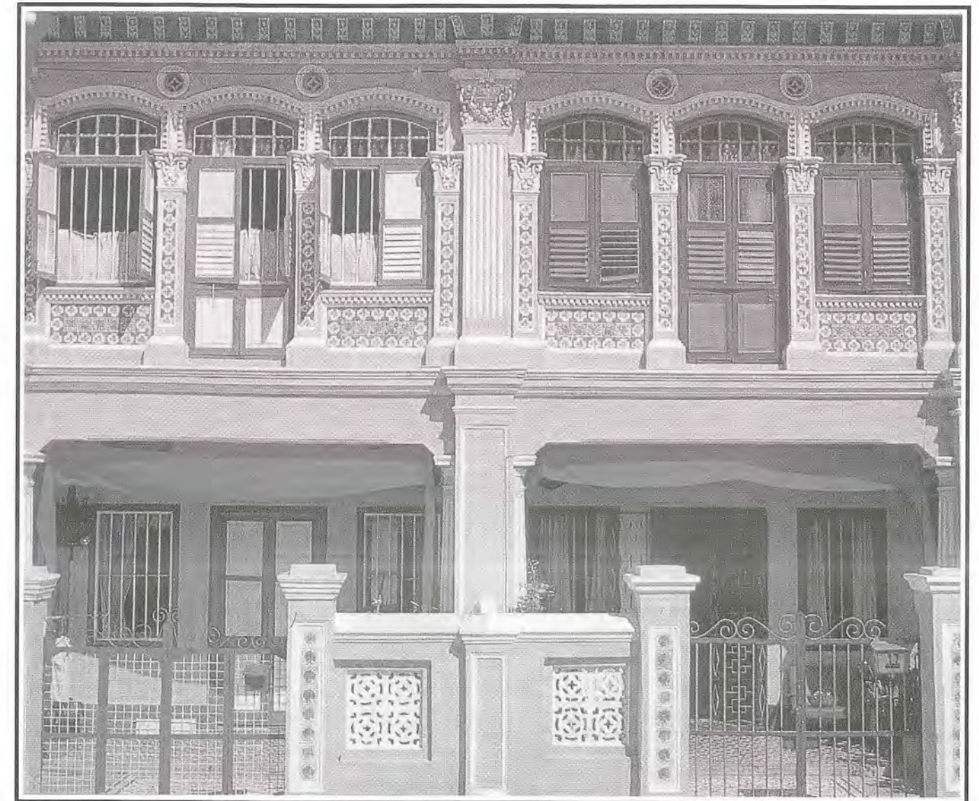
Fig 19: Careful restoration of the timber doors, French windows and casement windows enhances the overall character of the conservation shophouses.
