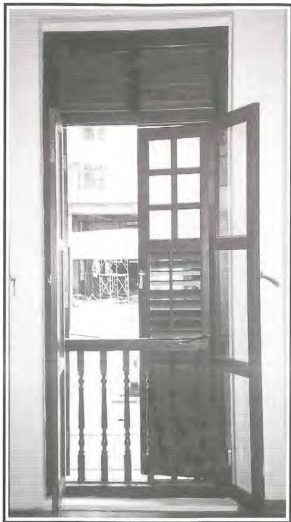
Fig 15: Intermediate rails of secondary windows matching those of the original casement and French windows.
