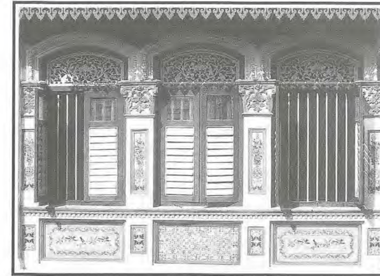
Fig 19: Careful restoration of the timber doors, French windows and casement windows enhances the overall character of the conservation shophouses.
