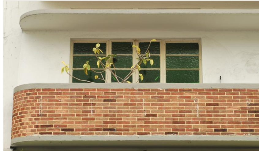
Balconies as a transitional space between the hot external climate and cool interior living space
