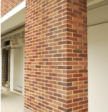
Fair-faced brickwork feature
