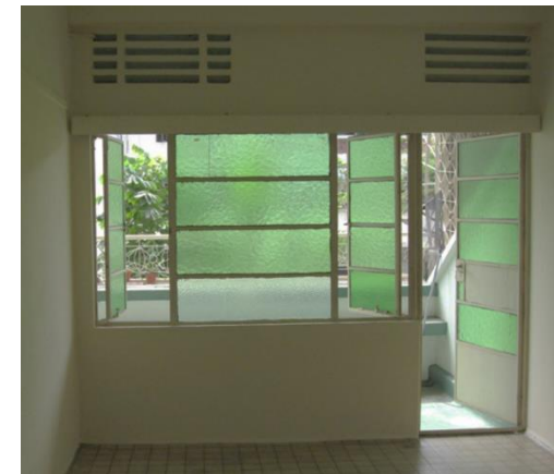
Tinted green glass windows protect occupants from the tropical glare and heat
