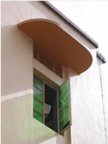
Curved sun-shades, and vents for natural ventilation
