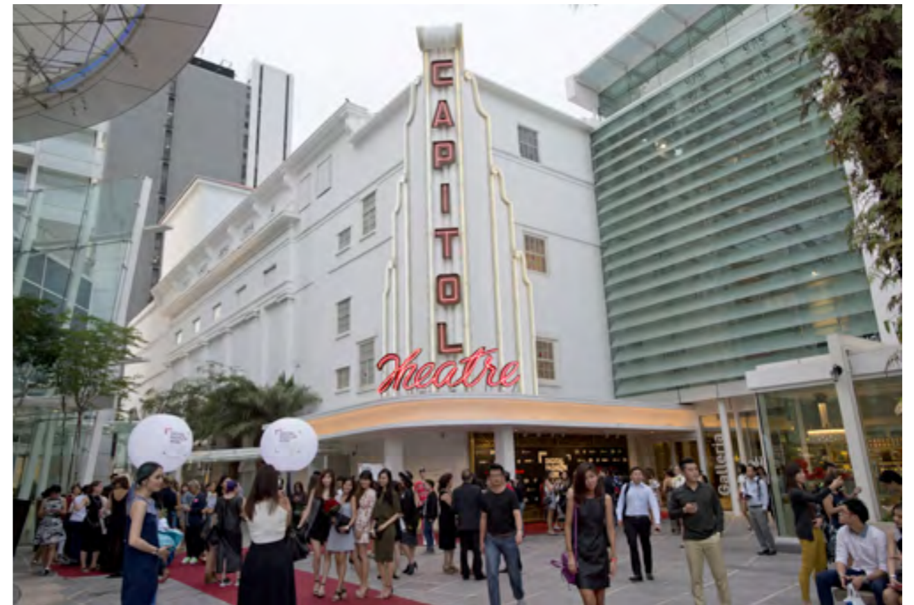
Above: The beloved Capitol Theatre has been brought back to glory, a result of four years of restoration work through strong collaboration between URA, Capitol Investment Holdings, Architects 61 and Studio Lapis.
