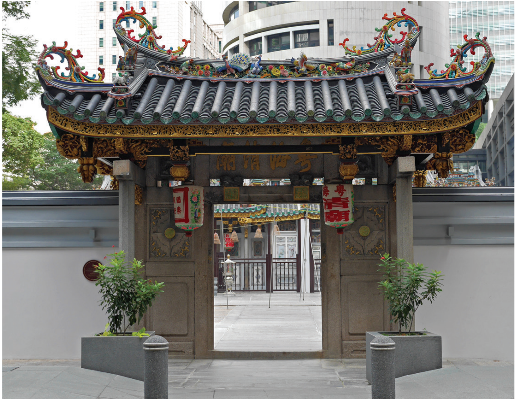
Yueh Hai Ching Temple garnered an URA Architectural Heritage Award for its masterful restoration
