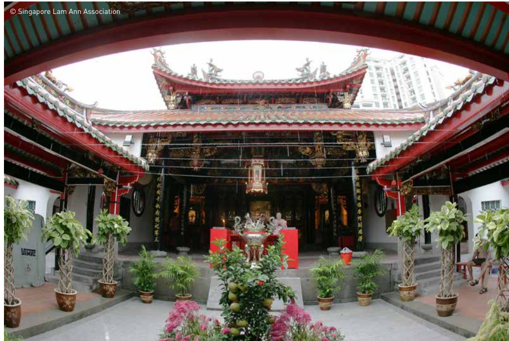
Thorough research and investigations helped restore the 100-year-old Hong San See Temple to its former glory
