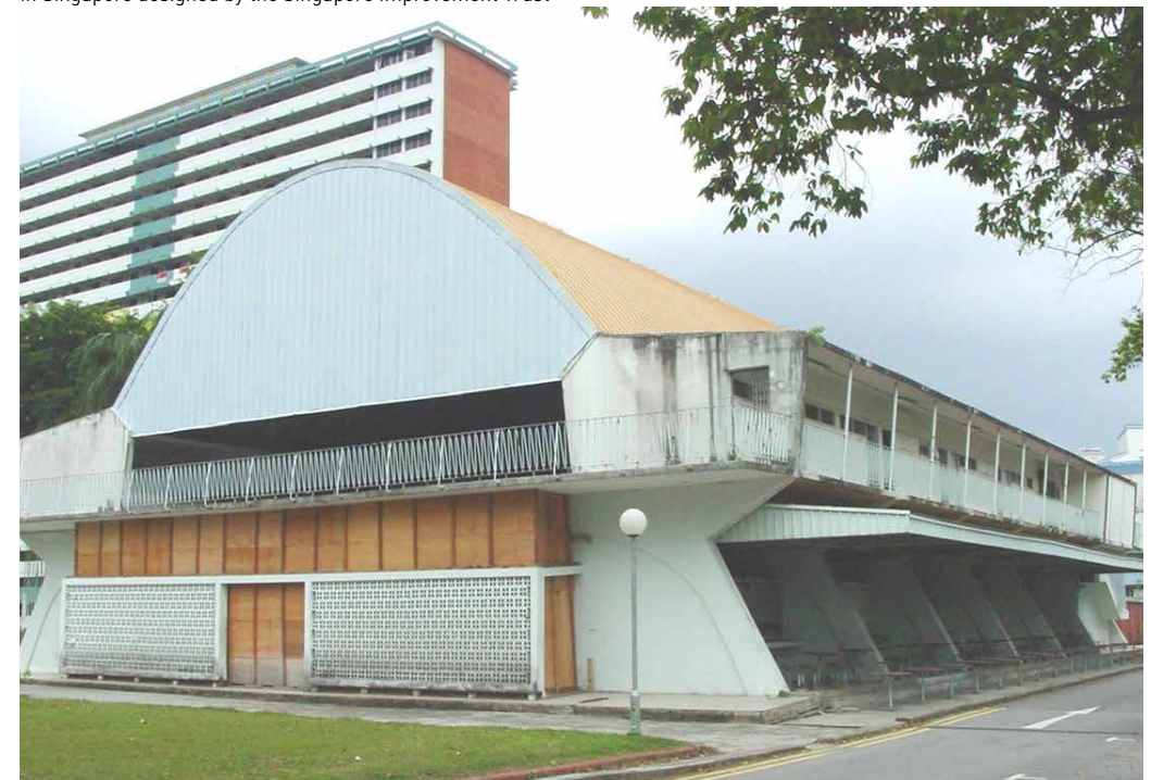
Opened in 1960, the former Commonwealth Avenue Market is the only remaining market in Singapore designed by the Singapore Improvement Trust
