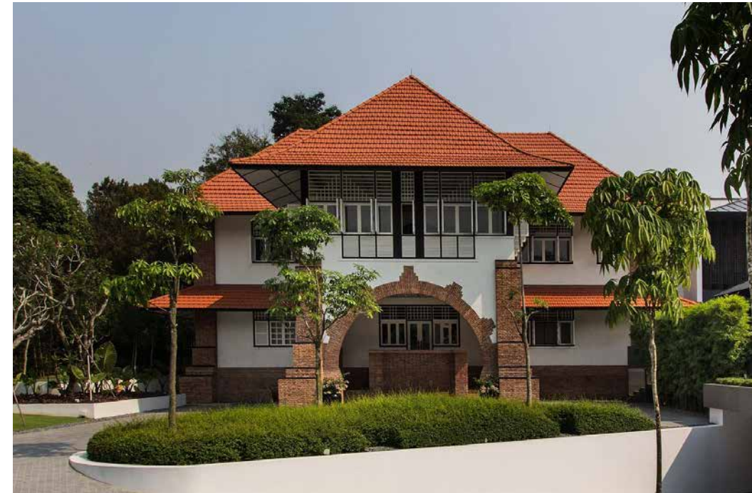
The signature Brewer exposed brick pillars at 5 Chatsworth Park were skilfully retained
