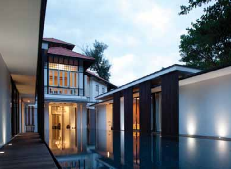
Above: A restored Black-and-White bungalow at 2 Cable Road
