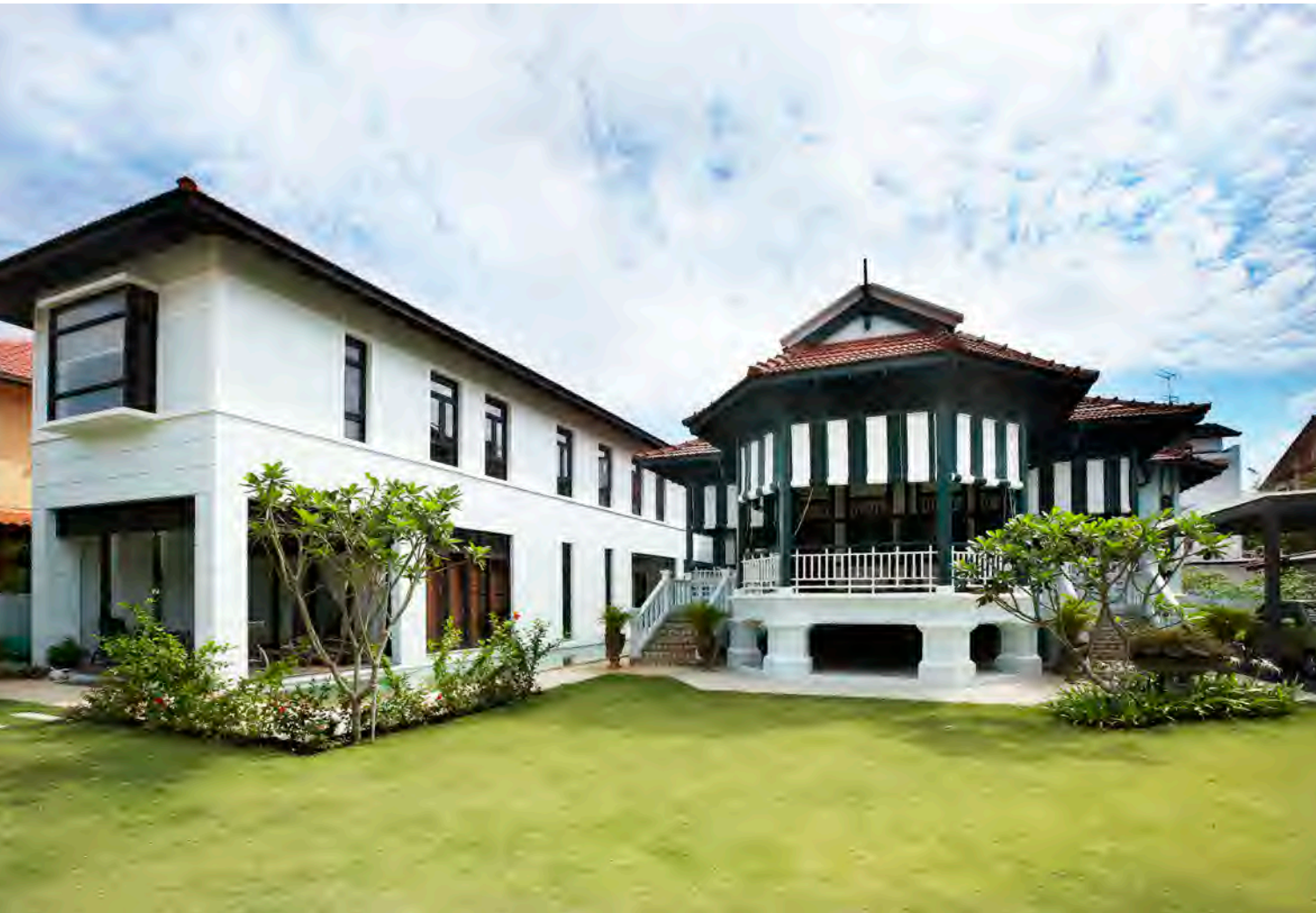
Refurbished Art Deco style bungalow at 25 Chapel Road
