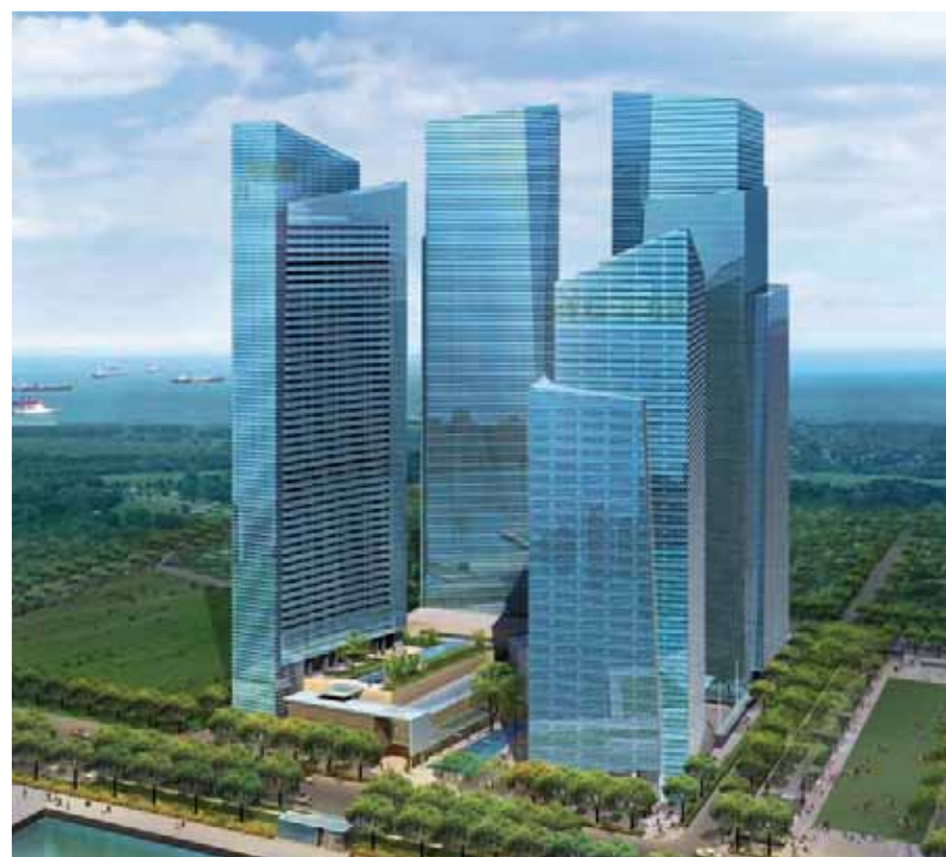
The Marina Bay Financial Centre will be part of the seamless extension of the CBD.
