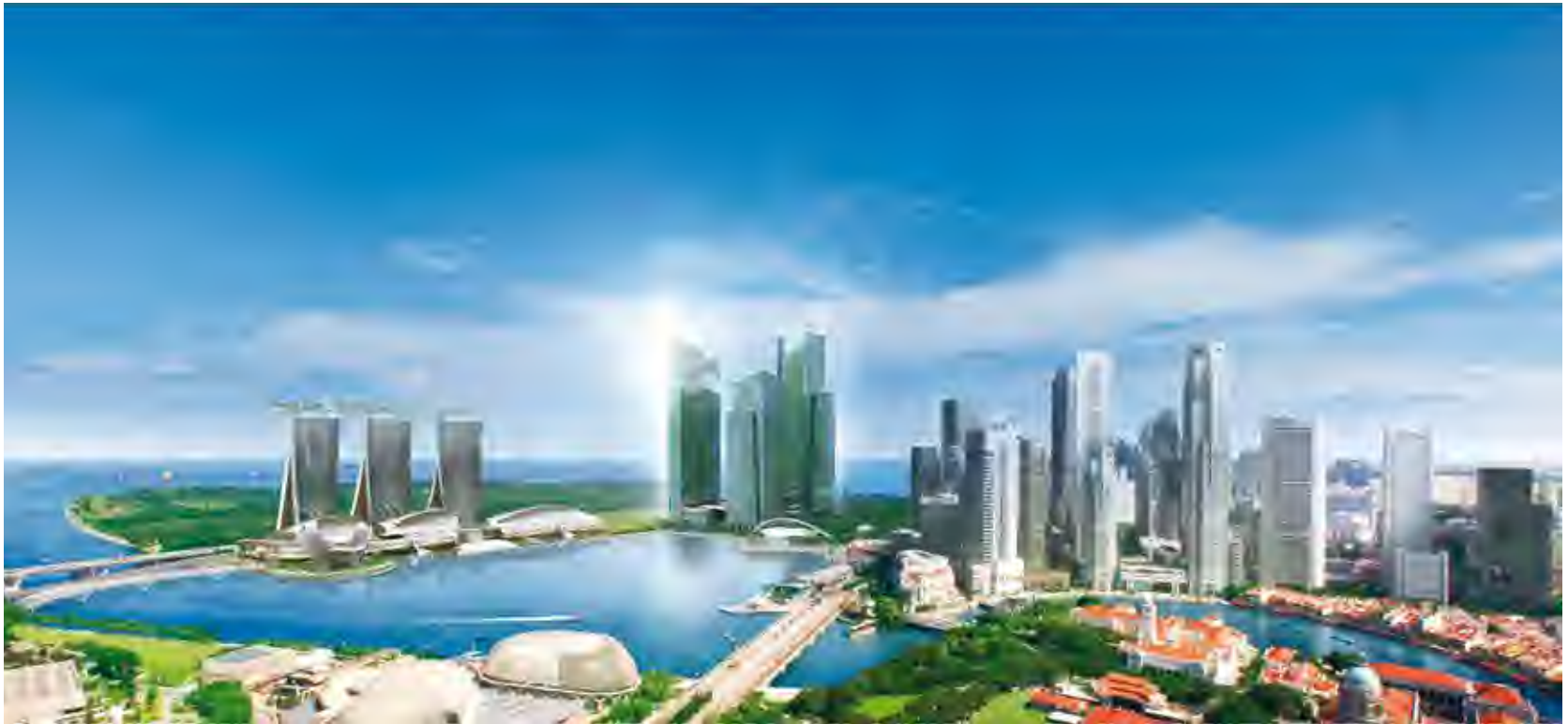
Redefining the Singapore skyline: The three soaring 50-storey hotel towers of the MBSIR and the MBFC's family of buildings placed to maximise views to and from the Bay.
