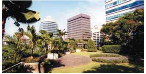
There is greater incentive to add pavilions on rooftop gardens like this on top of Shaw House, following URA's relaxation of guidelines.
