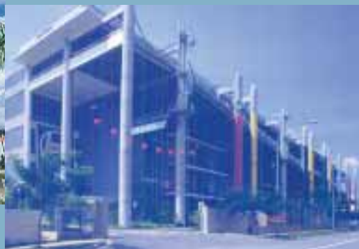
An example of a stack-up factory is the Ang Mo Kio Autopoint, a multi-storey car workshop.
