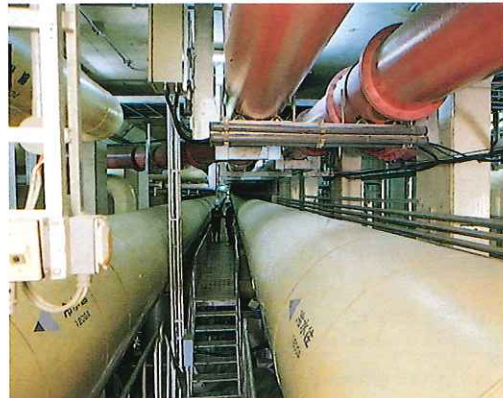
CSTs are already being used extensively in high-density urban areas in Japan and Europe. This is an actual CST in Yokohama, Japan.
