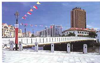
A fully restored Read Bridge
