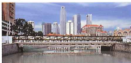
Ord Bridge undergoing restoration
