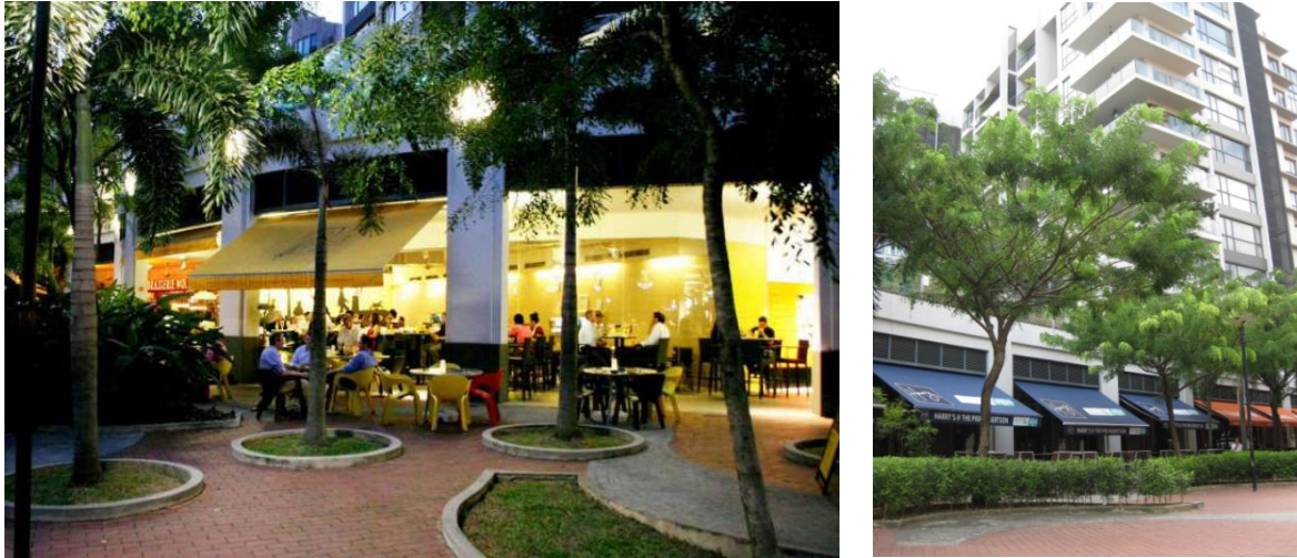
Figure 3-1: Awnings are to complement the scale and rhythm of the development façade, e.g. correspond to the column locations. Applicants should also seek clearances from SCDF on the location and extent of protrusion from the building façades.
