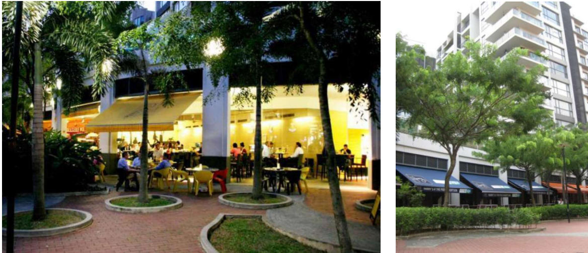
Figure 2-1: Awnings are to complement the scale and rhythm of the development façade, e.g. correspond to the column locations. Applicants should also seek clearances from FSSD on the location and extent of protrusion from the building façades.
