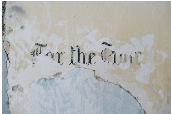
Following paint removal, a historically significant hand-painted sign was uncovered in the Church of St Teresa, indicating the original location of a donation box 'For the Poor'.
