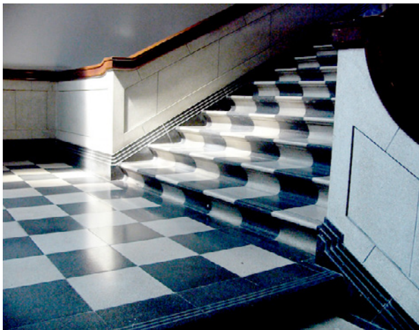
Above left: Black and white precast 'spuncrete' terrazzo tiles laid in checkerboard pattern, with special curved riser and grooved step riser units, likely custom-produced for the former Supreme Court (1939).
