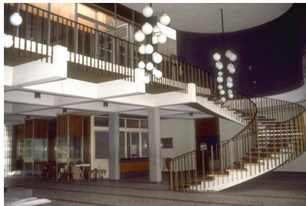
Open-well spiral stairway with curved reinforced concrete stringer supporting carpeted treads with brass balustrade, National Theatre (1963).
