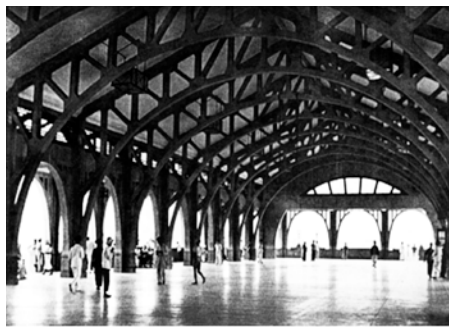
Left: Advertisement for ‘Spuncrete’ terrazzo products, a local innovation by the firm United Engineers Ltd. Middle: The old Clifford Pier was one of the earliest civic buildings in Singapore to use large slabs of ‘Spuncrete’ terrazzo flooring for its hard-wearing surface, ease of maintenance and attractive appearance. Right: Detail of precast terrazzo staircase treads at the former Supreme Court building. The side walls are lined with ceramic dadoes.
