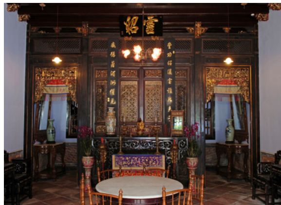
Left: Elaborate Chinese carved timber partition, or geshan, of a peranakan townhouse at 157 Neil Road. Right: Full-height timber lattice screen with top vents and double swing door ensures security and some privacy while facilitating ventilation.
