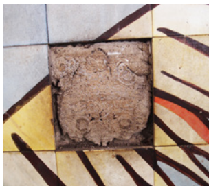
Ceramic tile debonded from bedding.
