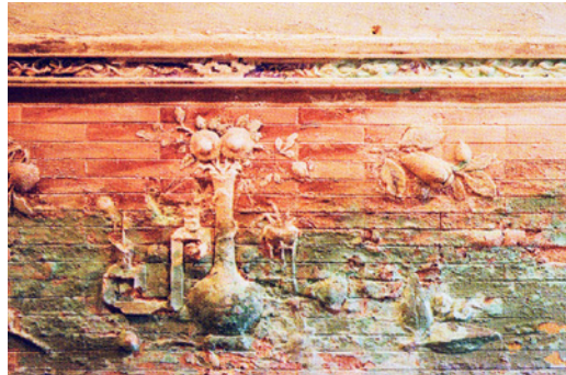
Deteriorated in situ decorative plaster dadoes, historic townhouses.
