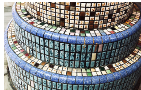
Left to right: Mosaic flooring accented with a grid of motifs, Church of St Bernadette (1959); Mosaic tiles with a raised embossed centre add visual texture and slip resistance, house at East Coast Road (1950s); Small mosaic tiles are used to wrap around curved surfaces such as this circular column in the Cundhi Gong Temple.
