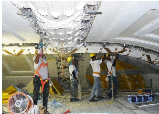
Restoration of reed motif moulding with design enhancement of its deteriorated borders, and reinstatement of rectilinear field mouldings.
