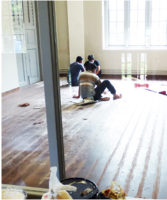
Left: Filling in the gaps between floorboards with filler strips and timber putty following reassembly. Right: Dismantling of timber strip flooring, revealing the joists beneath.
