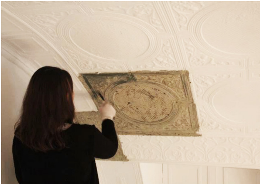
Trial paint removal of a metal ceiling panel using odour-free non-toxic biodegradable chemical stripper.
