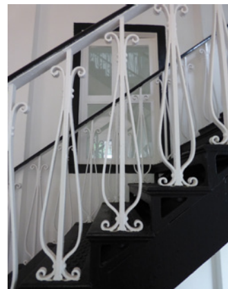
From left: Cast iron spiral staircase, National Museum of Singapore (1887), and riveted mild steel balustrade, 1920s colonial government quarter.
