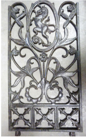
The fine details of the relief revealed, after removing multiple layers of coating from the overpainted baluster.
