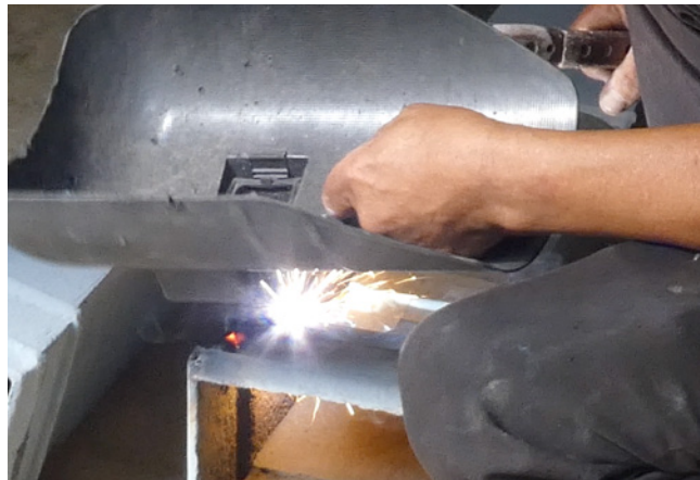
Hot repair of crack by welding.
