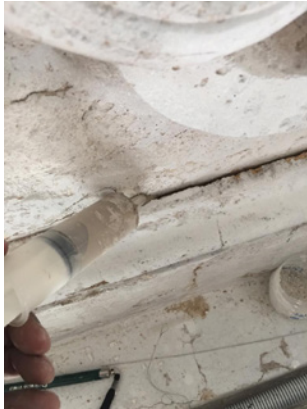
Debonding repair by injection.
