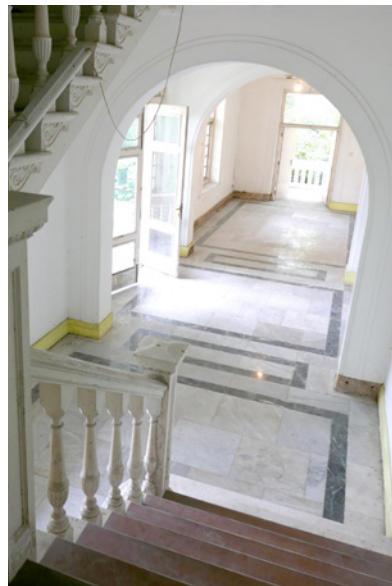
Above left: Marble flooring with dark green accents articulating the archways. Above right: Granite flooring, St. Andrew's Cathedral (1861).
