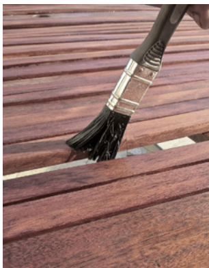
Revarnishing of wood as a regular maintenance practice.
