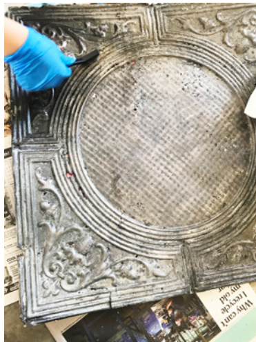
Trial application of coating on mild steel stamped metal ceiling panel with paint removed, beginning with a primer.
