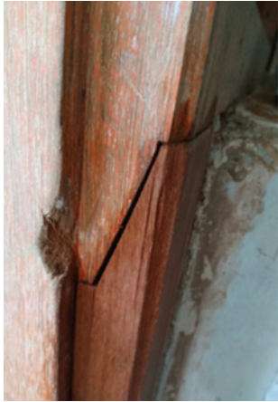
Timber-to-timber repair by splicing.
