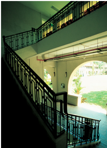
Above: Art Deco metalwork balustrade, Raffles College (1928). Left: Brass and bronze door accessories. Far left: Stamped metal panel dado, St Joseph's Institution (1910s).
