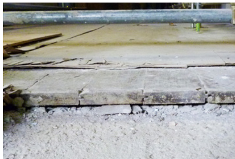
Left: Timber board flooring, Burkill Hall. Centre: Tongue-in-groove joints between floorboards revealed after dismantling of adjoining tiles. Right: Herringbone pattern parquet flooring.
