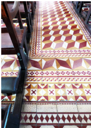
Cement tiles of a myriad of colours and geometric motifs line the nave of the Church of the Nativity of the Blessed Virgin Mary.
