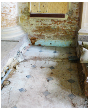
The original marble flooring at the Cathedral of the Good Shepherd, part of which can be seen in the archival photograph ( right ), was fully revealed after the latter-day mosaic flooring was removed ( left ). The marble tiles are one inch thick ( top ).
