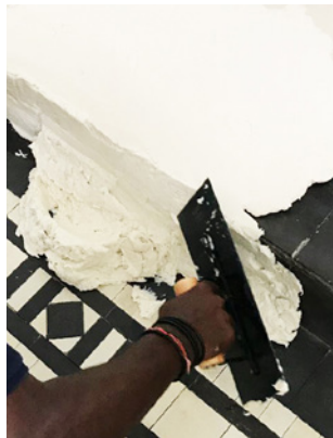
Desalination treatment by poulticing.
