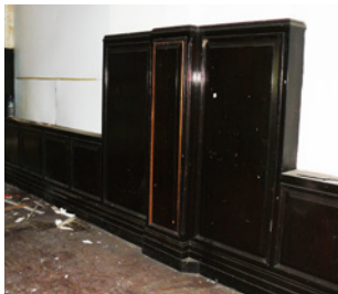
Historic carved timber dado panelling.
