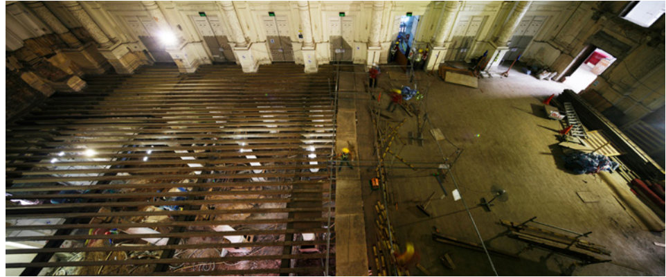
Left: Filling in the gaps between floorboards with filler strips and timber putty following reassembly. Right: Dismantling of timber strip flooring, revealing the joists beneath.
