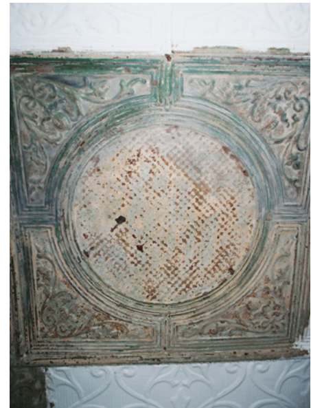
Trial paint removal of a metal ceiling panel using odour-free non-toxic biodegradable chemical stripper.
