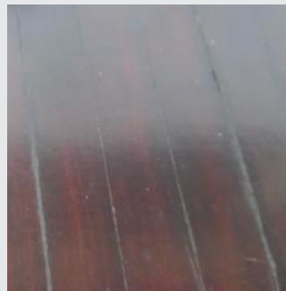
Timber floorboard (Verandah)
