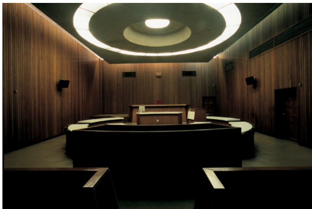
From top: Restored full-height moulded timber panelling, including cornices and architraves, 43 Amber Road (1900s); Grand timber coffered ceiling with moulded timber cornices, old Supreme Court (1939); Courtroom with timber strip wall cladding and built-in furniture, Subordinate Court (1975).
