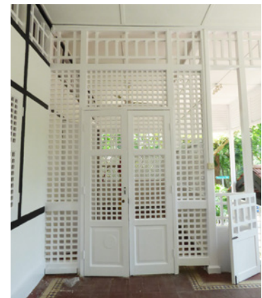
Left: Elaborate Chinese carved timber partition, or geshan, of a peranakan townhouse at 157 Neil Road. Right: Full-height timber lattice screen with top vents and double swing door ensures security and some privacy while facilitating ventilation.
