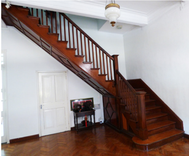
Left: Timber staircase with a bullnose starting tread and panelled undercroft. Centre & right: Ornate timber staircase with feature newel post.
