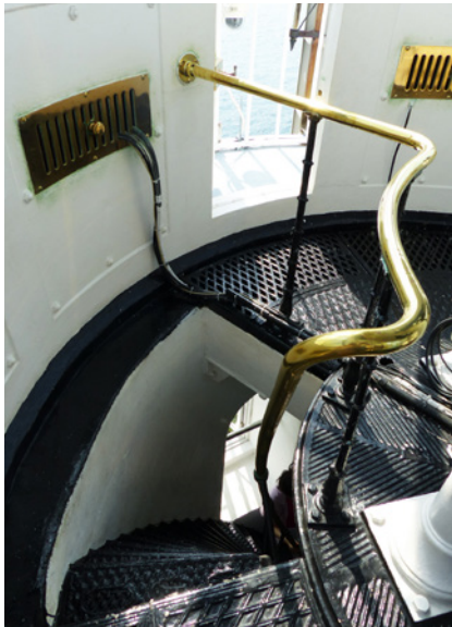
Iron spiral staircase with brass railing, and iron deck floor, Raffles Lighthouse (1850s).
