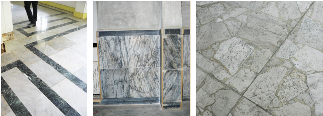
Left: Bichromatic stone flooring along the main hallway of a historic bungalow, comprising ‘field’ tiles in white Carrara marble, with border accents in dark green Serpentine marble. Middle: Book-matched Bardiglio Cappello marble dado in the former NAAFI Britannia Clubhouse (1953, aka NCO Club). Right: Detail of special Cocciame tiles comprising broken Travertino marble adhered onto a cement substrate, found in the former Trinity Theological College chapel (1969). The fragments are salvaged by-products of marble quarrying and cutting large blocks of natural stone.
