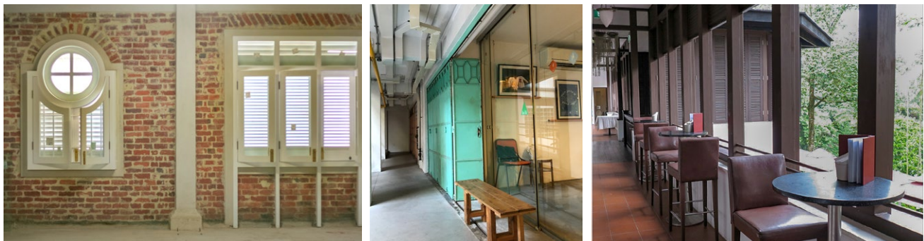
Left: Interior view of new timber frame secondary windows being installed, sensitively integrated with the historic window design. Middle: Frameless glass secondary sliding doors installed behind historic metal accordion gate. Right: New safety rail (horizontal steel bar) added to historic verandah timber frames of a restored bungalow due to the low sill height.
