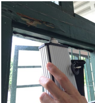
Timber resistograph carried out on window frame.
