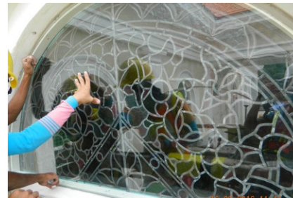
Installation of new external protective glass layer.
