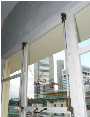
Original and replica mild steel pivoted windows at the former Brittonia Club (later NCO Club). Reinstatement using replicas was done for window locations where the original had been demolished.
