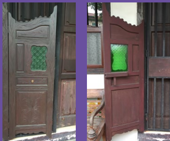
Exterior- and interior-facing sides of a pintu pagar with coloured embossed glazing panel.
