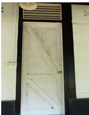
Board and batten door
