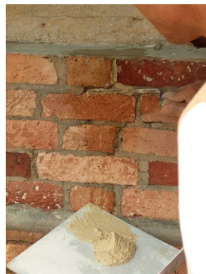
Repointing trial for fairfaced brick masonry wall.
