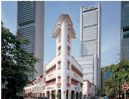
Circular Road shophouse (1938)
