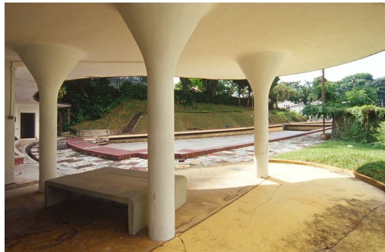
Flared mushroom columns and cantilevered flat slab roof in reinforced concrete, former Yan Kit Swimming Complex (1952).
