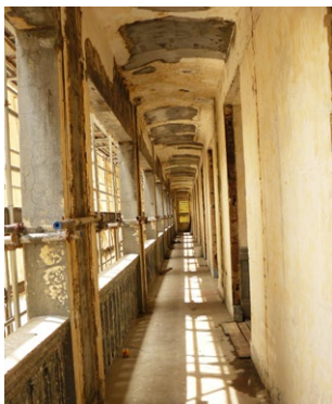
From top: Concrete patch repair – removal of affected concrete cover to expose rebar for cleaning and treatment, before patching with compatible mix.
