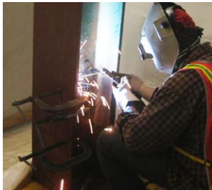
Welding repair of steel column base.
