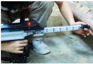
Above: Specialist carrying out resistance drilling measurement on a timber structural member.
