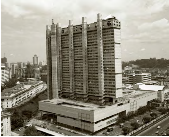
Left: People's Park Complex (1973) - the podium is clad with rusticated concrete panels, designed such that each could be lifted manually by one or two workers. Right: Singapore Polytechnic at Prince Edward Road (1972) - concrete panels are used as infills for the structural frame. Slender sunshading fins express the buildings structural and design datum.
