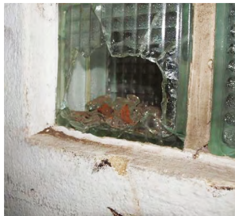
Right: Broken glass block. Far right: Painted surface on a glass block.
