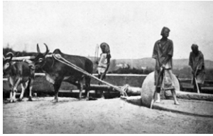
Mortar Mill at the grounds of Government House during construction, 1860s.
