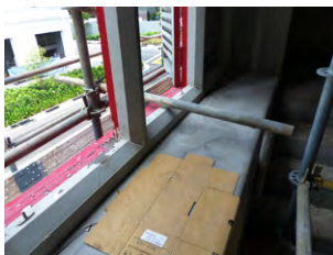
Above: Temporary structural propping for facades. Left: Scaffolding and props erected without impacting facade fabric and finishes – anchorage achieved by padded clamping and utilising existing openings.
