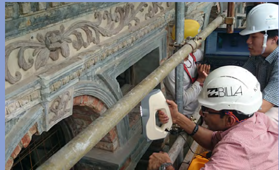
Ways to document ornamental plaster for restoration - Top: Profile gauge measuring devices. Above: Handheld 3D scanning device.
