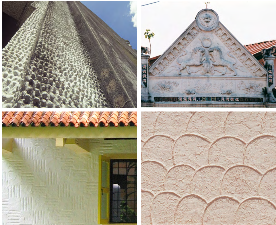
Clockwise from top left - hand-tooled ornamental plasterwork found at: former Ford Factory (1941); shophouse pediment (c.1890s); St. Andrew's School (1940); former Anglo-Chinese School Cairnhill campus (1928)
