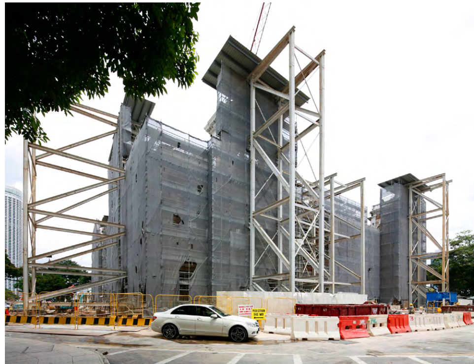
Above: Temporary structural propping for facades. Left: Scaffolding and props erected without impacting facade fabric and finishes – anchorage achieved by padded clamping and utilising existing openings.
