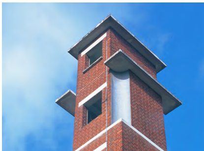
SERANGOON FIRE STATION
