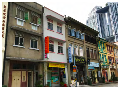
BUKIT PASOH SHOPHOUSES
