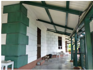
The Raffles Lighthouse (1855), built entirely in granite blocks, with quoin detailing.
