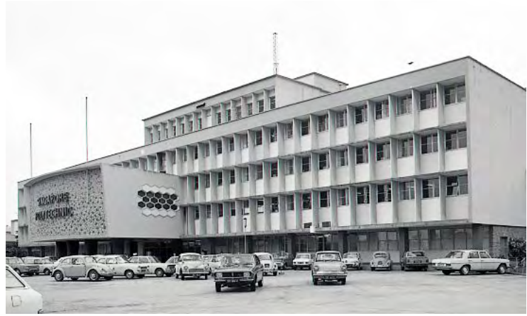
Left: People's Park Complex (1973) - the podium is clad with rusticated concrete panels, designed such that each could be lifted manually by one or two workers. Right: Singapore Polytechnic at Prince Edward Road (1972) - concrete panels are used as infills for the structural frame. Slender sunshading fins express the buildings structural and design datum.
