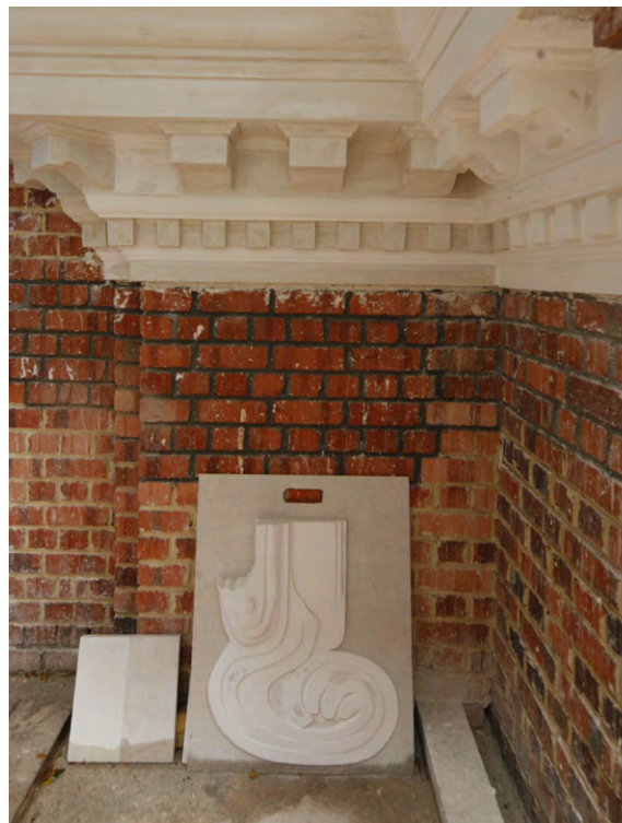
Mock-up for ornamental plaster mouldings at Victoria Concert Hall.
