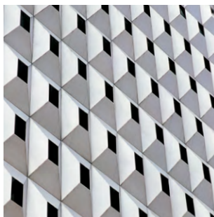
Metal eggcrate clad over an older shophouse facade instantly lends the building a dignified appearance.
