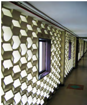
Left: People's Park Complex (1973) - the podium is clad with rusticated concrete panels, designed such that each could be lifted manually by one or two workers. Right: Singapore Polytechnic at Prince Edward Road (1972) - concrete panels are used as infills for the structural frame. Slender sunshading fins express the buildings structural and design datum.
