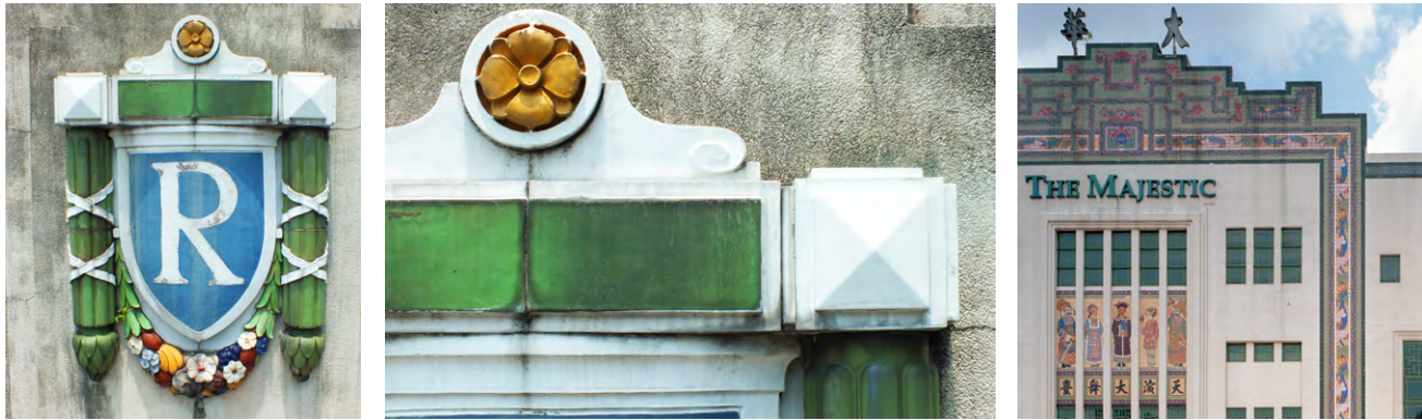
Left, Middle: Customised glazed terracotta units were tailored to create a set of four coat-of-arms on the Tanjong Pagar Railway Station main facade, featuring the initials of the Federated Malay States Railway. Right: Majestic Theatre facade
