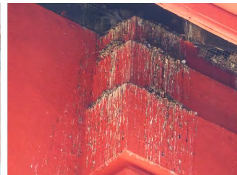
Left: Wasp infestation on fairfaced brick facade. Right: Accumulated bird fouling.
