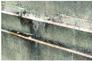
Top: Severe efflorescence accumulating on the Shanghai plaster surface.
