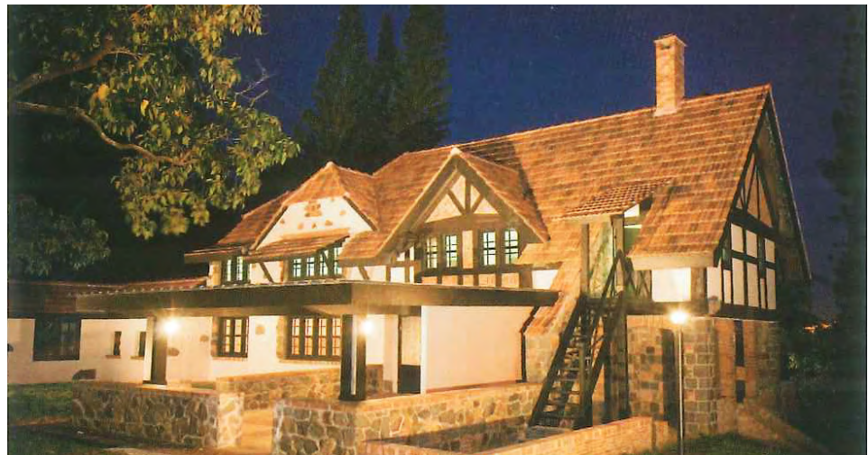
The fairfaced stone masonry walls on House No. 1 at Pulau Ubin, originally the house of Chief Surveyor Langdon Williams, displays the impeccable quality of the granite quarried from the island.
