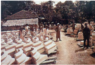
Top: Cav Rudolfo Nolli and his masterpiece – the Shanghai Plaster facade ornaments at the old Supreme Court (National Gallery today). Above: Nolli and his Foochow artisan team in his casting yard at 47 Scotts Road.
