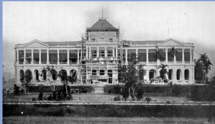
Government House nearing completion, 1869.
