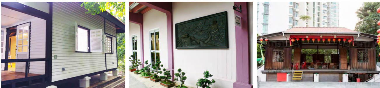
Left: Overlapping wooden boards on the facades of the former farmhouse at Dairy Farm Road. Middle: A rare existing example of timber sidings used for institutional buildings, at the Pasir Panjang English School. The timber lightweight infill spans between RC columns which are expressed on the facade. Right: Tan Kong Tian Temple Stage at Jalan Kebaya (1919). The timber structure sits on masonry piers, raised above ground moisture.
