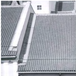
New flashing lining the junction between roof covering and partywall.
