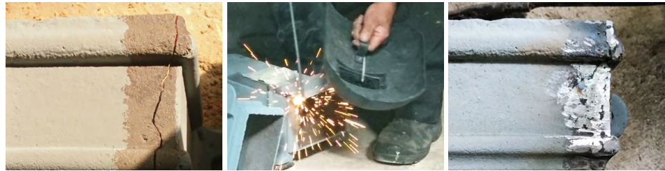
Crack repair by welding for cast iron downpipe.
