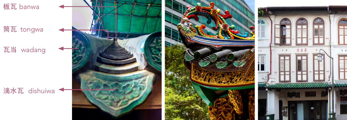
Left: Different tile types in the Chinese roof tiling system as seen at Wak Hai Cheng Bio. Right: First storey awning with green glazed Chinese tiles and granite bracket at a shophouse along Telok Ayer Street.
