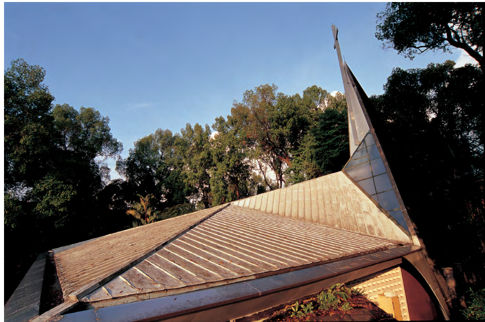
Maris Stella Chapel features an expressive roof composed of a few simple pitched roof planes with sheet metal roofing, constructed in situ with hand-crimped standing seams that are folded flat at the edges. A skylight is incorporated as part of the roof design.
