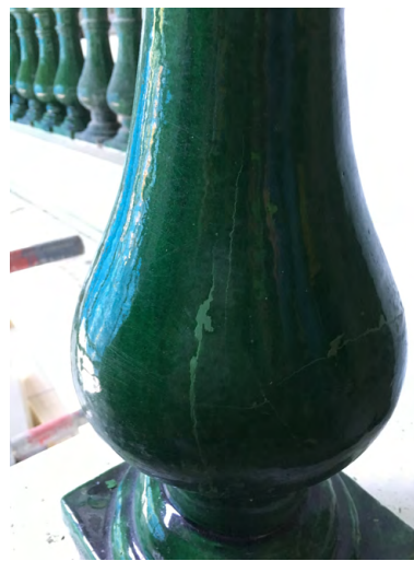
Patching of fine cracks on green glazed bottle balustrade.
