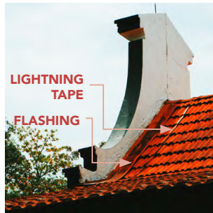
Roof accessory elements to check during maintenance inspection.
