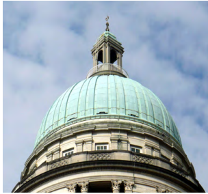
Patinated copper dome roof at the former Supreme Court.
