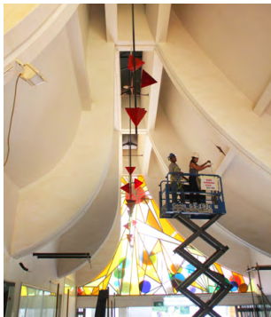
Ceiling inspection using elevated access equipment to reach high areas.
