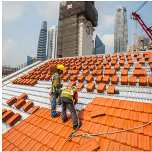
Interlocking clay tiles laid on metal battens atop secondary metal roof.
