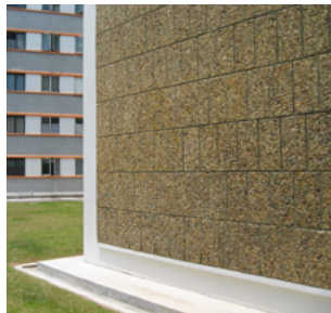
From top: precast vent block screen and exposed aggregate panelling at Old Kallang Airport Estate embody the 'architecture of economy' approach to design in resource-scarce postwar Singapore. Building materials were used in experimental and innovative ways that did not compromise on aesthetics.
