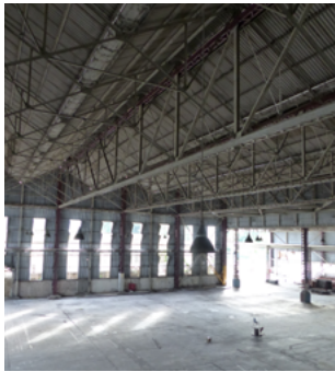
The soaring interiors of the Kallang Airport Hangars, one of the largest structures of its kind in the region when completed.
