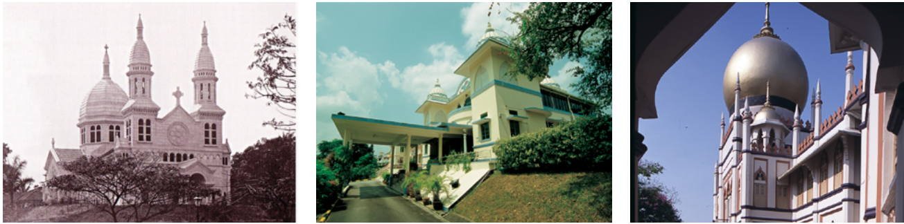
From left: St. Teresa Church (1929), Ramakrishna Mission (1940s–50s), Sultan Mosque (1932).
