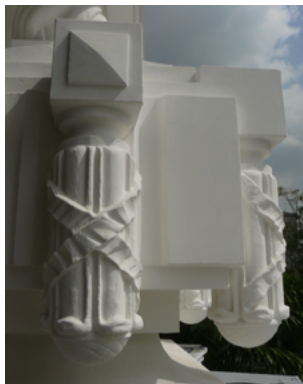
Pre-cast ornaments in the form of reed bunches adorn the Capitol Building.
