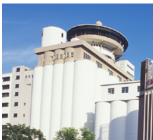
The distinctive concrete silos at Prima Flour Mill.
