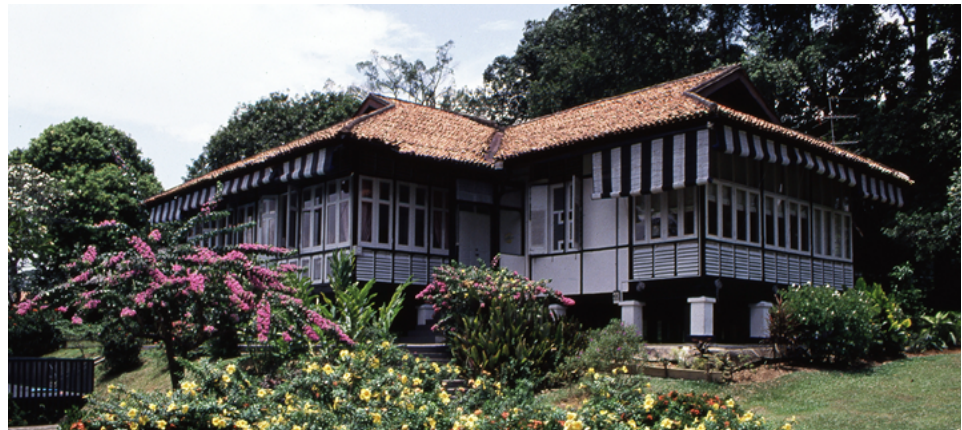
From top: Inverturret at Gallop Road, a plantation villa-type design with the upper floor raised high for surveillance of the grounds; A black and white bungalow at Dalvey Estate, with distinctive black timber frames.
