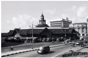
One of the earliest preserved examples of civic buildings include Telok Ayer Market, established in 1825, moved and rebuilt in cast iron in 1894.
