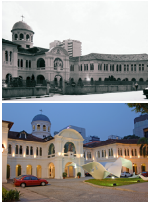
Originally a school, the former St. Joseph's Institution building on Bras Basah Road has been adapted for reuse as the Singapore Art Museum.
