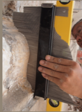
LEFT: A profile gauge for recording simple profiles on cornices. ABOVE: Replica created from a silicone mould.
