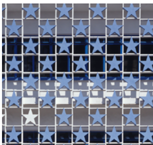
Lea Hin was one of the early local mild steel component manufacturers. Its headquarters building is clad in a distinctive sunshading screen of mild steel grid and stars.
