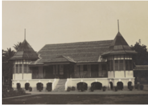
An example of a Malay Bungalow with low piers and an entrance stairway.
