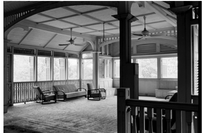
Left: Raising houses on high piers also aided ventilation. Right: A breezy upper floor verandah sitting room decked out in carved timber elements, with a porous enclosure of louvered French windows, balustrade and top vents.
