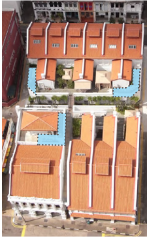
Discreet placement of M&E equipment on the roof terraces.
