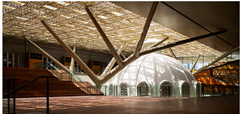
Left: Sunlight is filtered through perforated metal screens installed below the glazed panels, supported on a few slender 'tree columns'.
