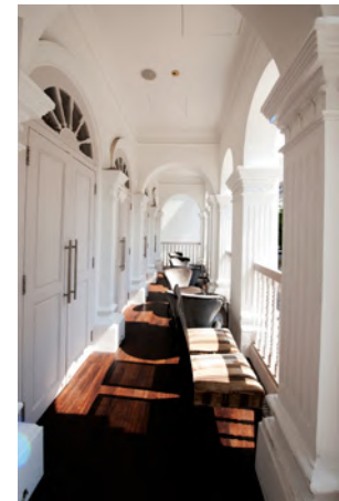
Left and middle: Second storey dining hall with air-con units, service pipes and trunking decanted outside. Outlet penetrations are discreet and carefully coordinated with the interior historic elements. Right: Verandah outside the dining hall, with a false ceiling concealing the FCUs.
