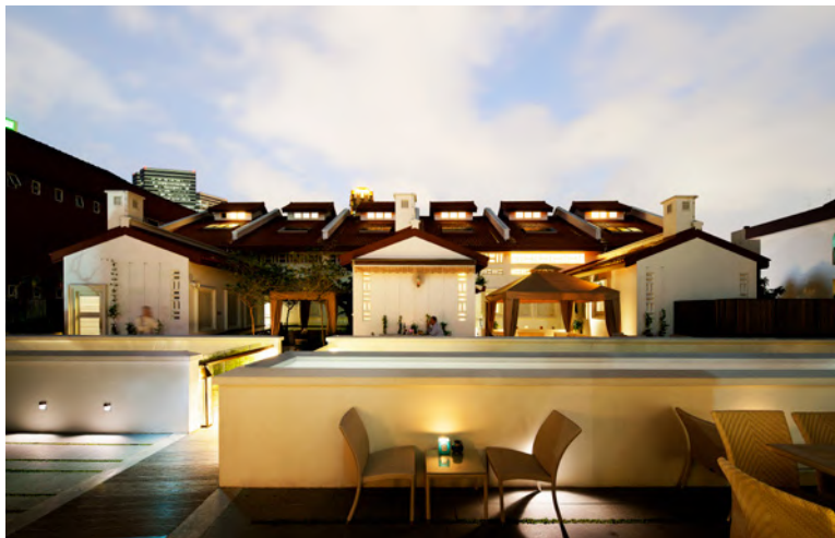
Above: New roof terraces connect the two wings while serving as a dining patio and open-air lounge.
