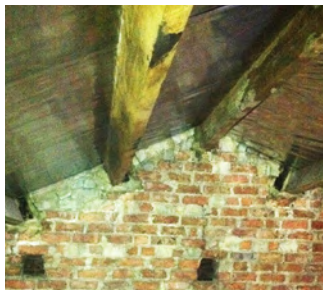
Left: Historic timber roof purlins being restored in situ as interior features. Middle: A new lightweight steel frame of beams, joists and slender columns extending to the first storey being installed for the new attic. Right: Completed new attic deck and restored historic timber purlins, exposed by installing roof insulation and ceiling board between members.
