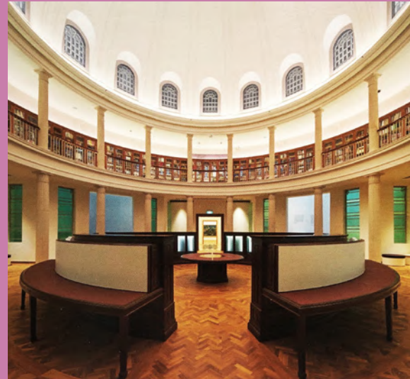
The restored Rotunda Library. New secondary anti-blast windows that match the historic design are installed at the clerestory lights of this space.
