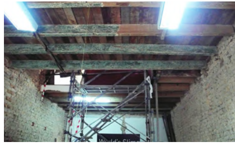
Above left: Originally exposed timber floor concealed at the five-foot way. Above right: Restoring timber joists found intact above false ceilings.
