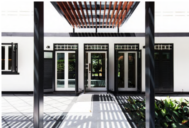
Left: Incorporation of Low-E glazing and security card reader on the secondary layer of like-for-like replacement fenestrations.
