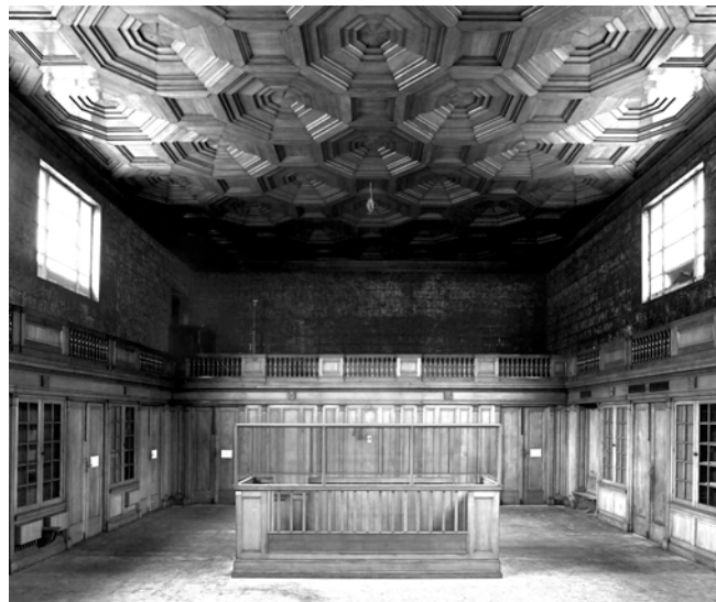
Left top: One of the courtrooms undergoing restoration. The mezzanine was originally lined with pivoted mild steel windows providing the interiors with daylight illumination.
