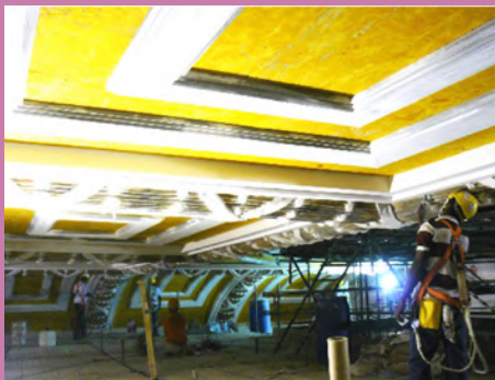
Left and right: Missing architectural features such as the ceiling coffers were reinstated using acoustic panelling whose design matched the historic details.
