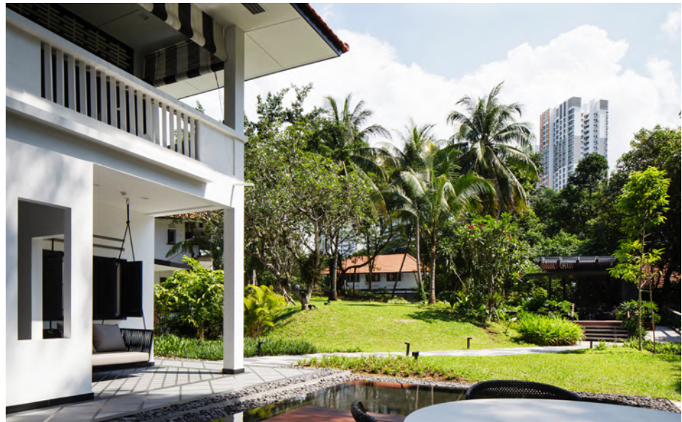
Historic residences are adapted for commercial institutional use, with seminar rooms for structured learning as well as informal interaction spaces.
