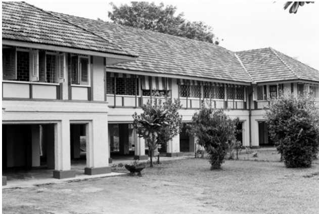
Left: Raising houses on high piers also aided ventilation. Right: A breezy upper floor verandah sitting room decked out in carved timber elements, with a porous enclosure of louvered French windows, balustrade and top vents.
