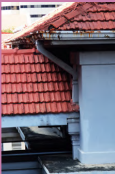
Left: Badly deteriorated historic cast iron rainwater goods . Middle and right: Restored historic rainwater gutter and rainwater downpipes along all facades and internal courtyards of the building .
