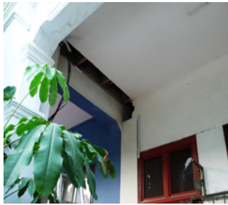
Above left: Originally exposed timber floor concealed at the five-foot way. Above right: Restoring timber joists found intact above false ceilings.
