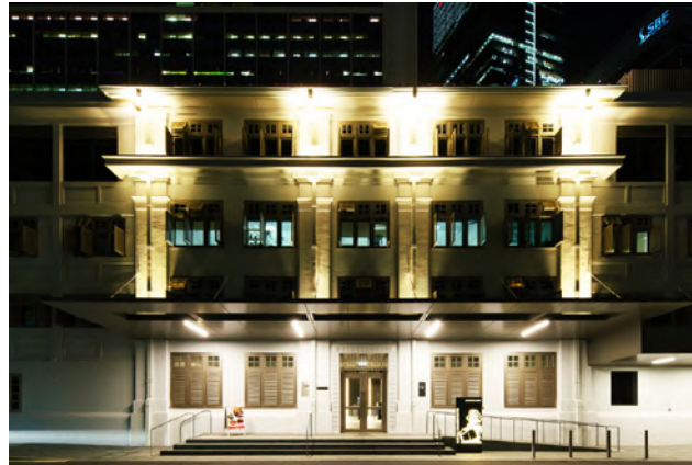
Main vehicular entrance at the rear facade of the building, with steps and ramps leading into the raised main lobby.
