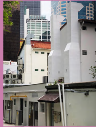
Neatly integrated kitchen exhaust flues on the rear service blocks of shophouses.
