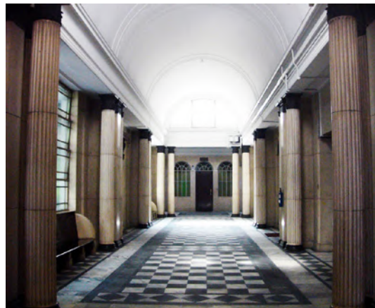
The clerestory lights facilitate daylighting and natural ventilation of the deep plan interiors, with dramatic illumination highlighting the corridor junctions, vaults and reflecting off the mother-of-pearl terrazzo finishes.
