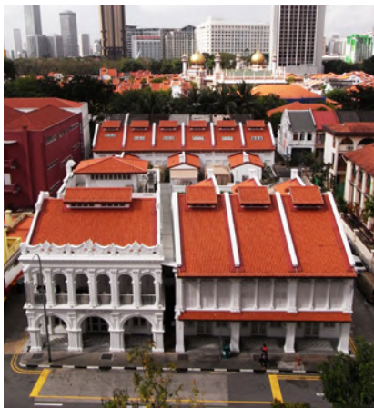
New jackroofs are introduced, in keeping with the architectural vocabulary of townhouses/shophouses.
