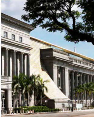
The new glazed canopy drapes over the new main entrance to the NGS atrium.
