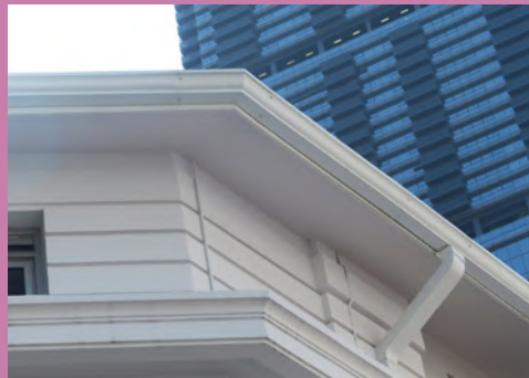
Left: Badly deteriorated historic cast iron rainwater goods . Middle and right: Restored historic rainwater gutter and rainwater downpipes along all facades and internal courtyards of the building .
