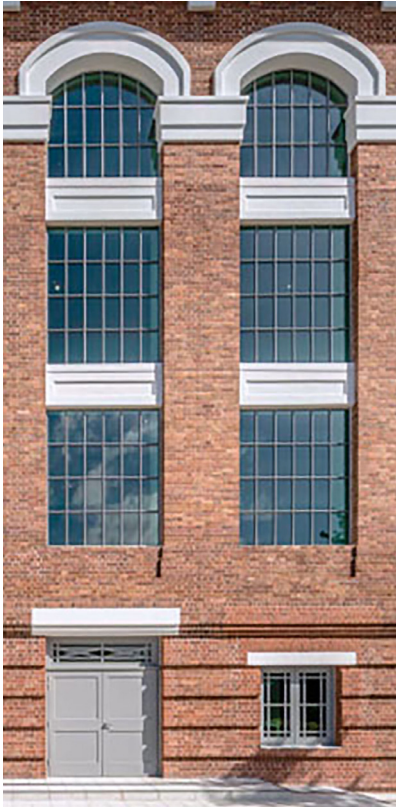
Reinstated mild steel window frames
