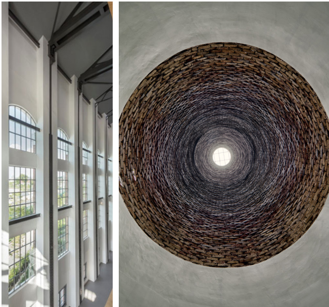
Original elements of steel and brick structures revealed
