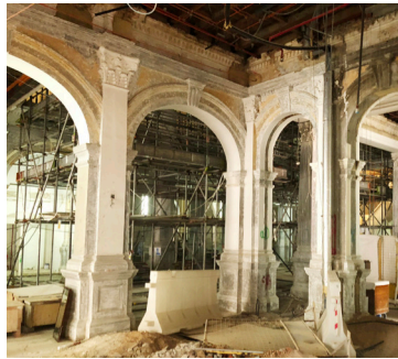
Cast iron stripped for repair
