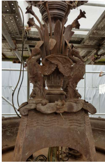
Cast iron stripped for repair
