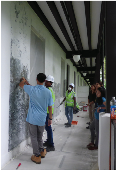
Thorough treatment for moisture
