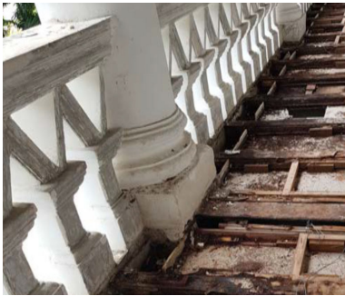
Careful examination carried out to guide restoration approach
