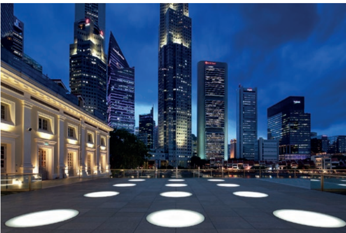
New roof terrace allows for appreciation of heritage facade and skyline
