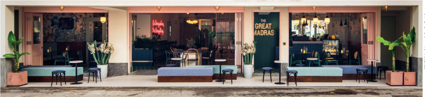
Open concept on first storey lobby has added life to the street
