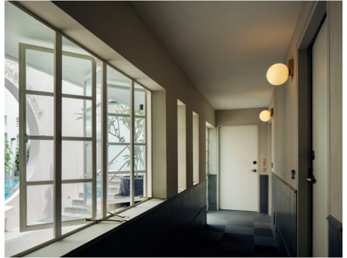
New mild steel windows along airy corridors
