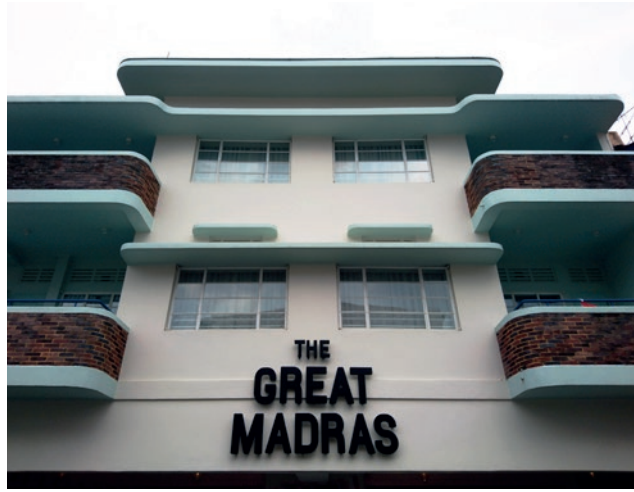
Restored facade with new Art Deco colour scheme
