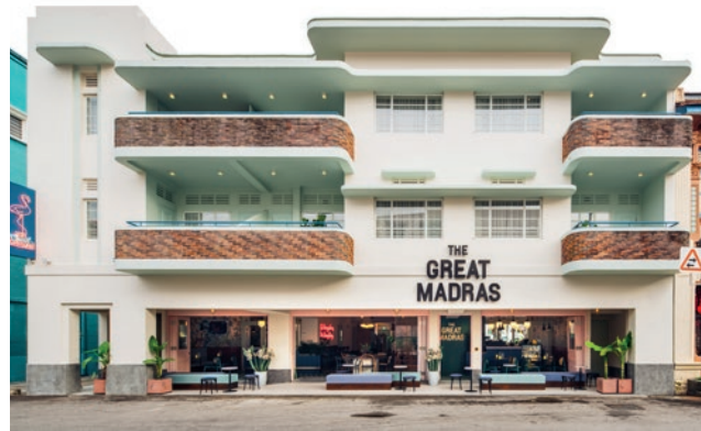
Former Singapore Improvement Trust flats in the Little India Historic District
