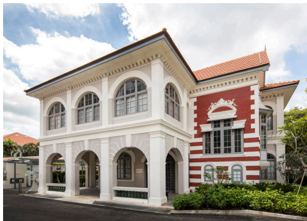
Front facade of the Rectory
