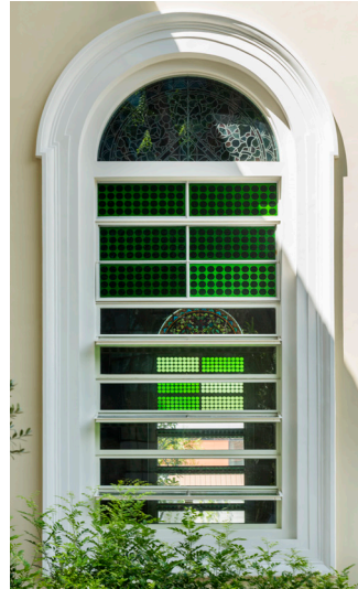
Original mild steel pivoted window with green glass
