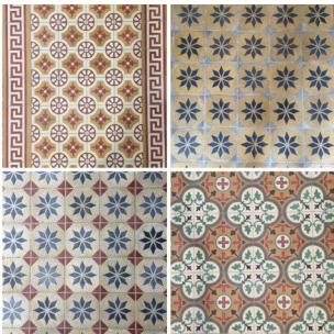
Original encaustic floor tiles in the Rectory
