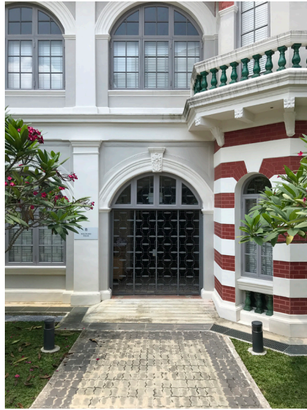
Rear entrance of the Rectory
