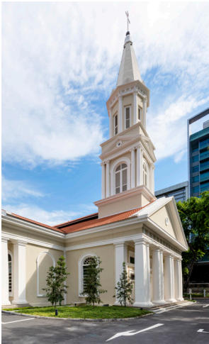
Steeple and the reinstated East portico
