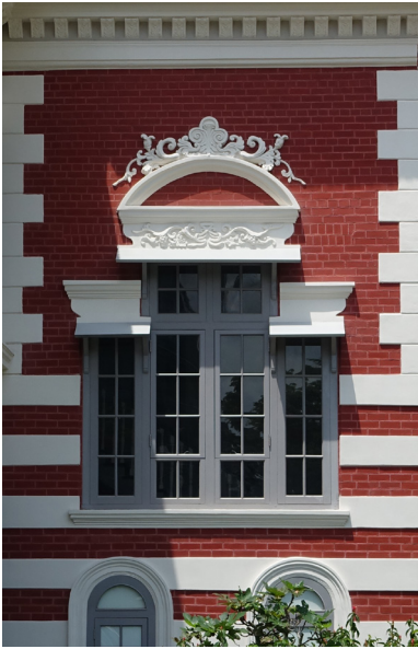
"Blood and bandage" facade reinstated
