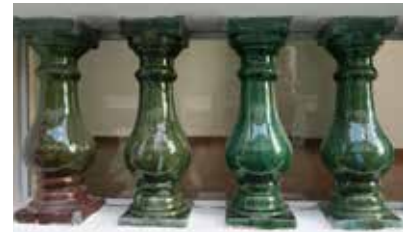
Glazed balustrades cleaned
