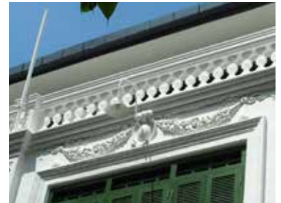
Carefully cleaned plaster details
