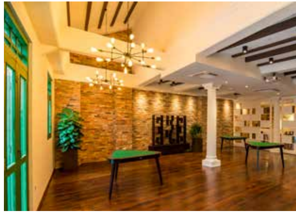
Bricks were salvaged and reused in the interiors
