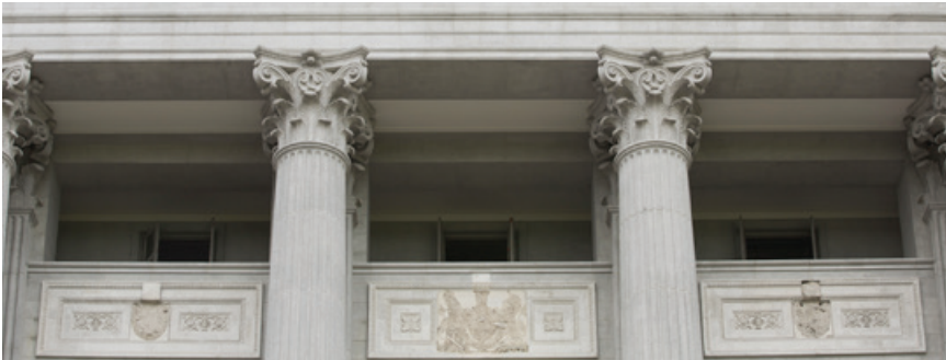
Shanghai plaster Corinthian capitals of former Supreme Court
