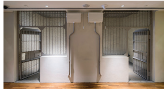
Jail cells at former Supreme Court restored and adapted into gallery space
