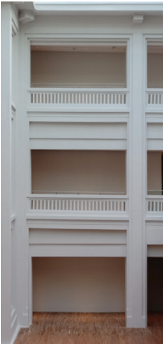
Courtyard façades of the former City Hall retained
