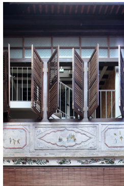
Timber window shutters
