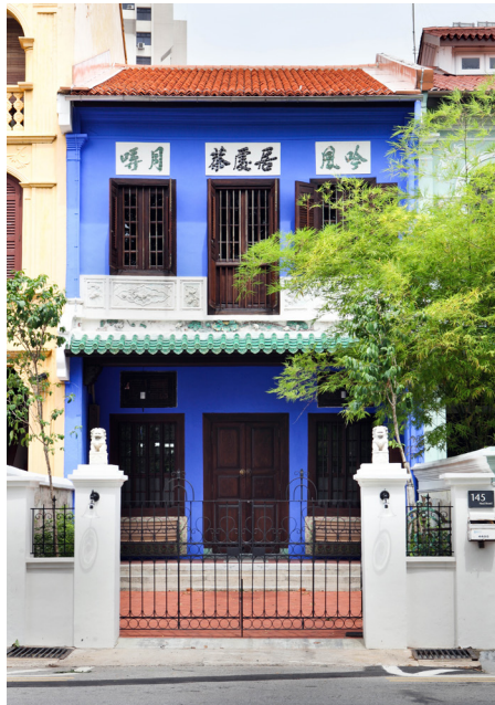
Transitional-Style Shophouse restored and repaired in vintage-inspired blue
