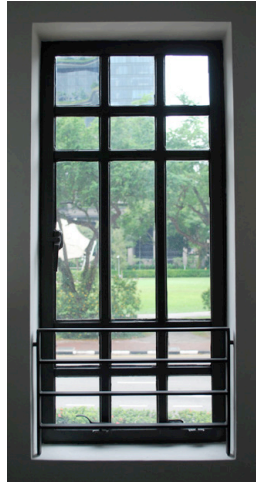
Mild steel windows reinstated
