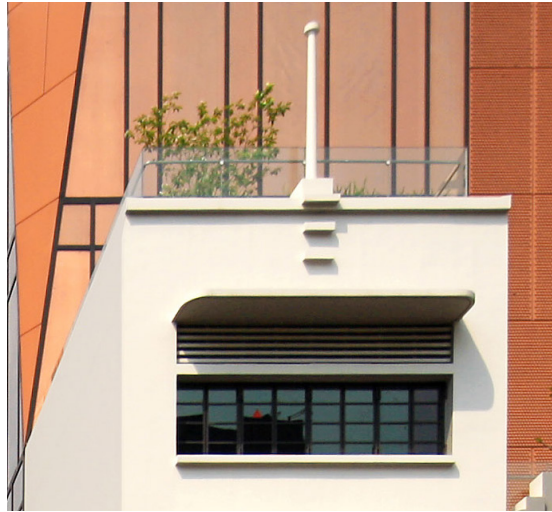
Concrete flagpole and canopy of Modern shophouse
