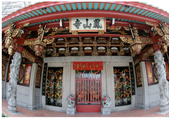
Original spatial quality of front entrance reinstated
