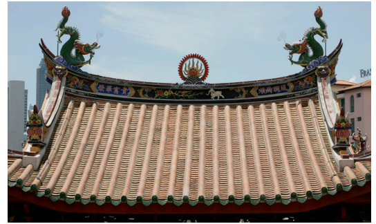
Original roof with natural clay tiles and green glazed eaves and dragon motif finials
