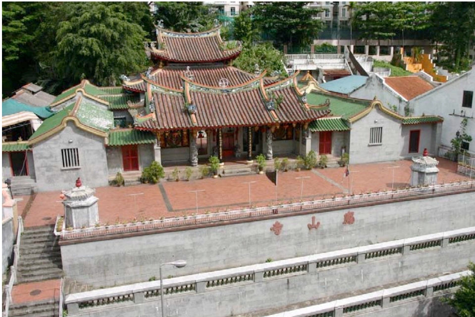
Pre 2006–2009 Restoration Overall View Selected Pre-Restoration Photographic Documentation, dated 2004 (Photo Credit: Patrick Goh)
