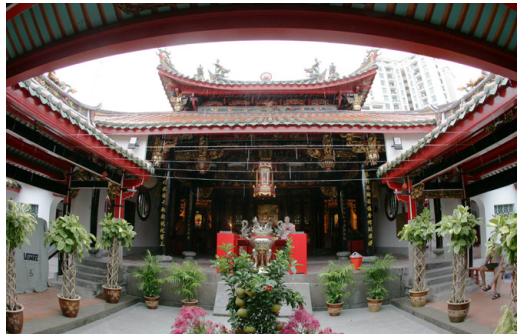
Restored Main Hall with double-eaves gable and hip roof
